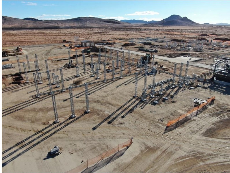
Figure 5-3: A Switching Station under construction 20 .
