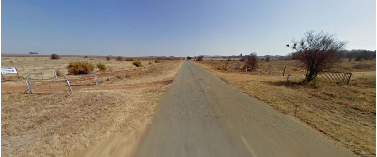
Figure 7-16: A view of the Road S 171. The road will provide direct access to the project site of the proposed project.
