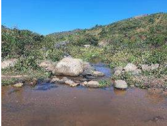
Downstream photo of a reach of SE-Transitional River-468 at the location of a causeway road crossing.
