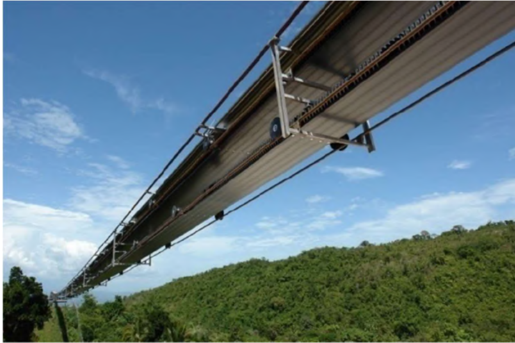
Figure 3. Typical RopeCon Section
