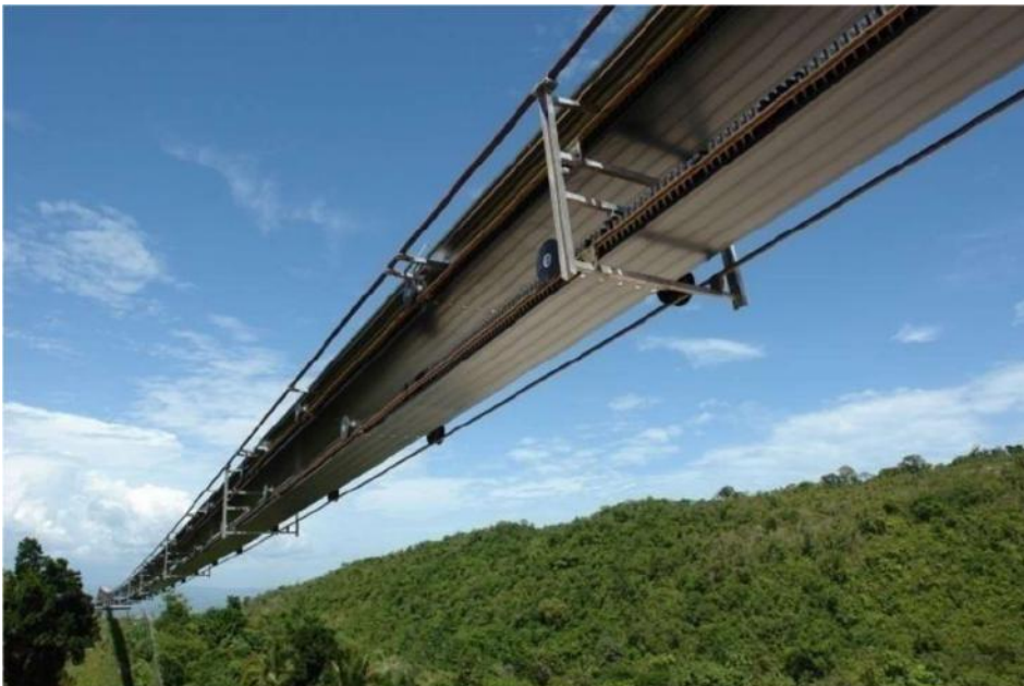
Figure 3-3 Typical RopeCon Section
