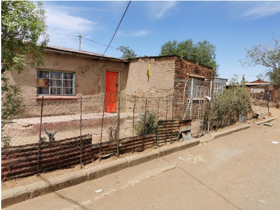
Figure 13: View of one of the houses in Itumeleng where maildrops were distributed.
