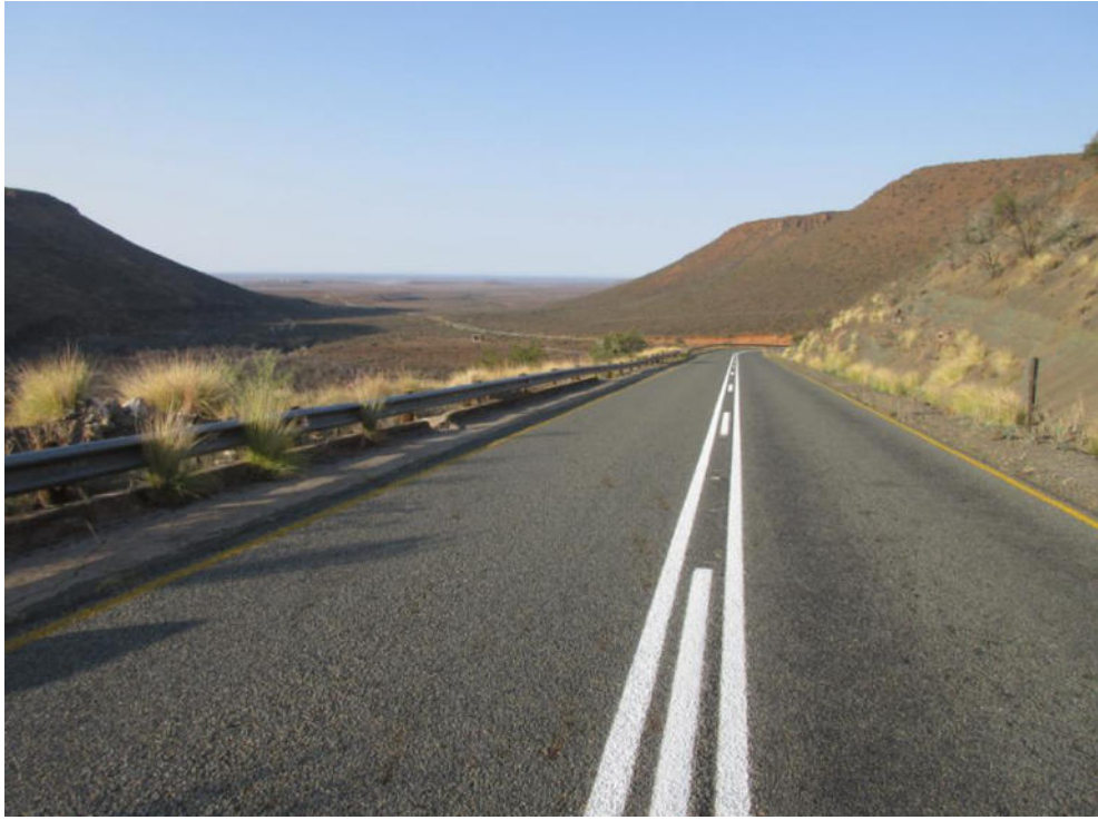
Figure 7 - Paved Section of R381
