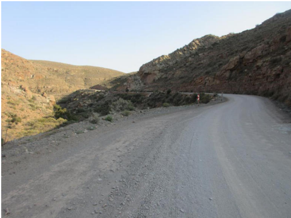
Figure 8 - Unpaved Section of R381
