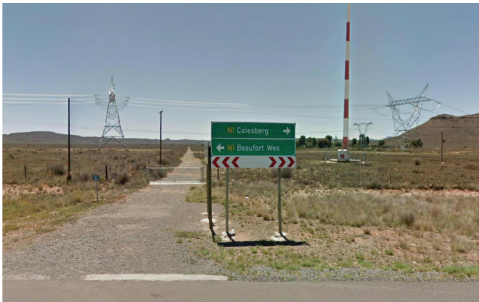
Figure 15 - OP09225 at the intersection with the N1
