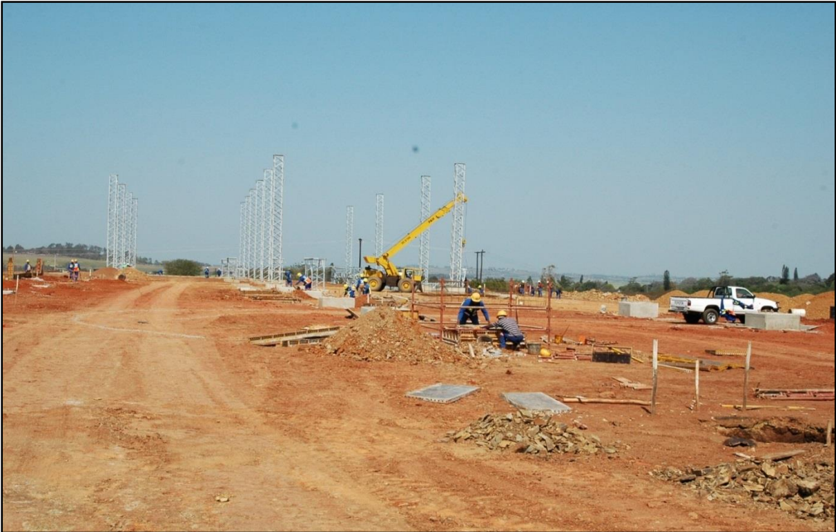
Plate 5: Erection of steelworks
