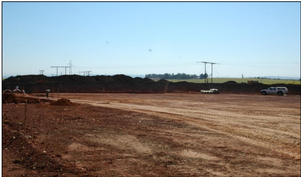
Plate 2: Levelling and terracing of the surface
