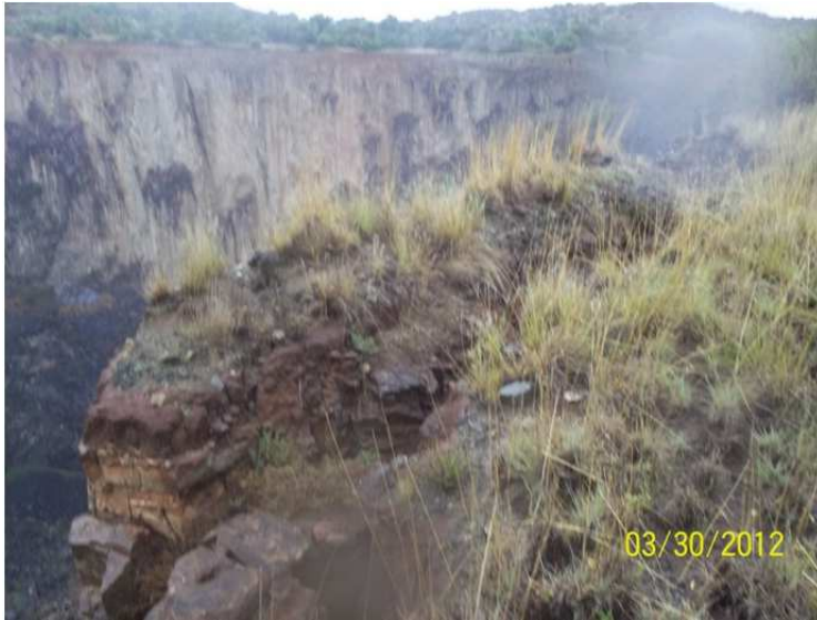
Figure 4-10 : Block of material about to fall into the pit
