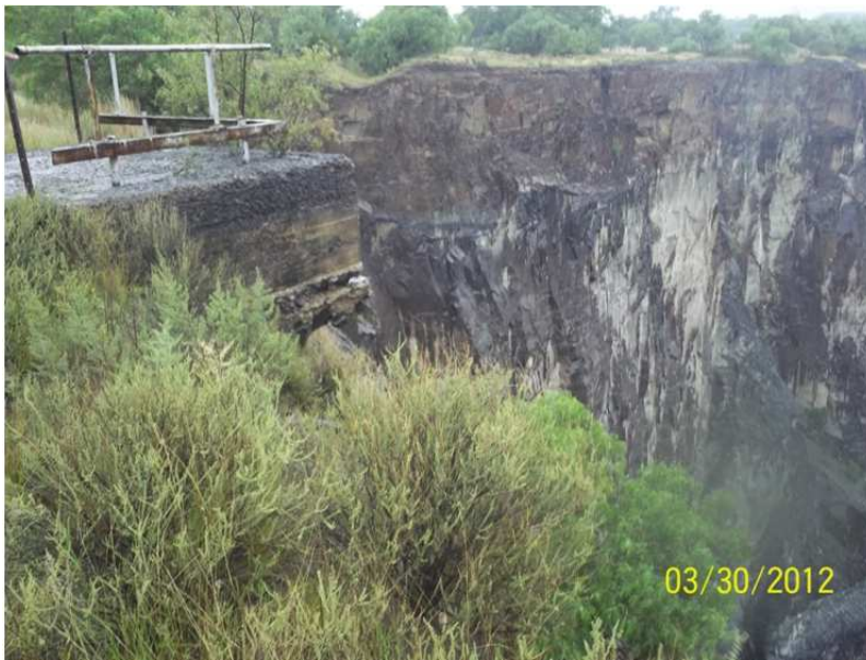
Figure 4-8: Condition of the outlook position
