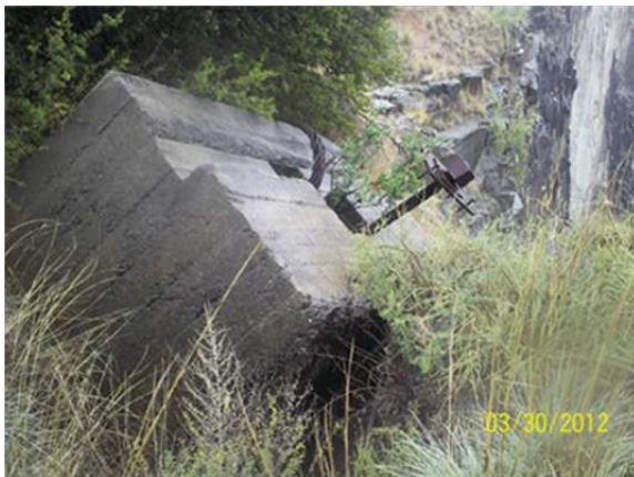
Figure 4-9: Old undermined installations
