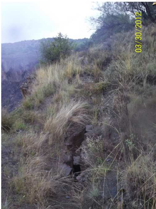
Figure 4-11 : Numerous cracks at a distance of between 5m and 10m from the edge of open pit
