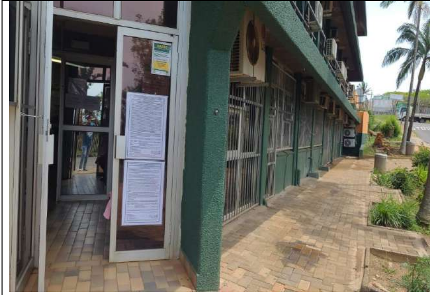
Site notices placed at the main entrance to Empangeni Clinic dated 27 October 2022.
