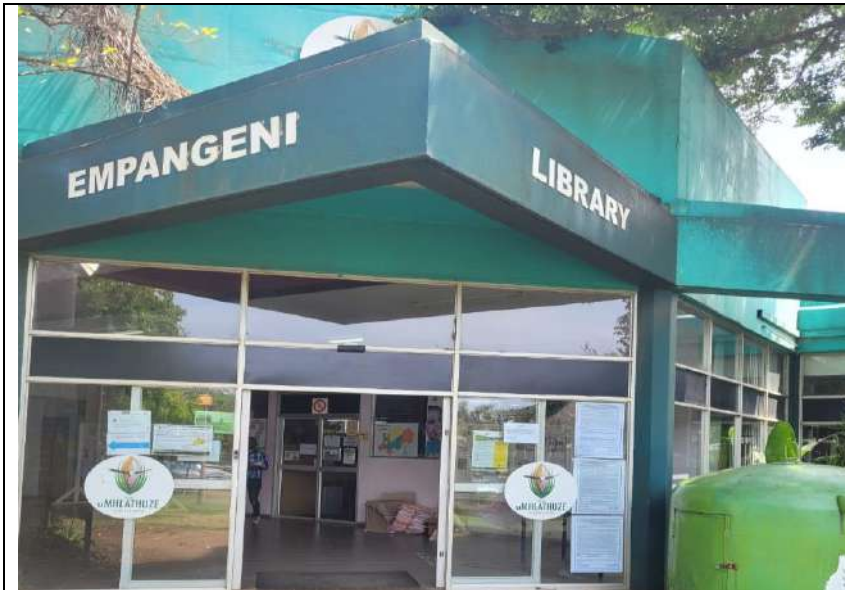
Site notices instated at the entrance to the eMpangeni Library dated 27 October 2022.
