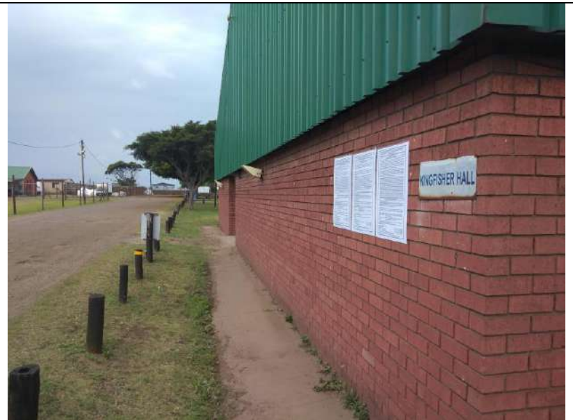
An alternative view of the site notices placed at Zululand Chambers dated 24 October 2022.
