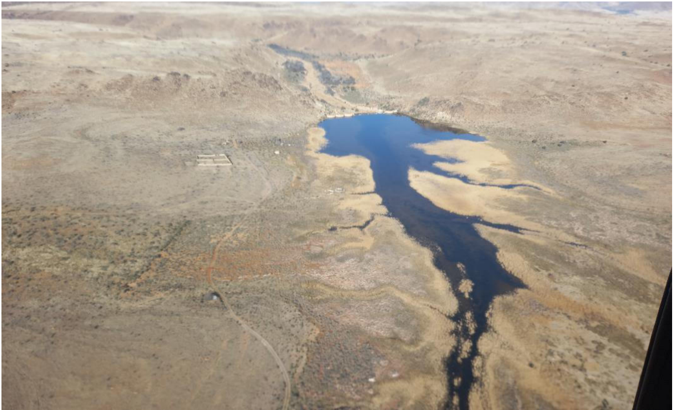
Figure 3: A large dam in the assessment corridor
