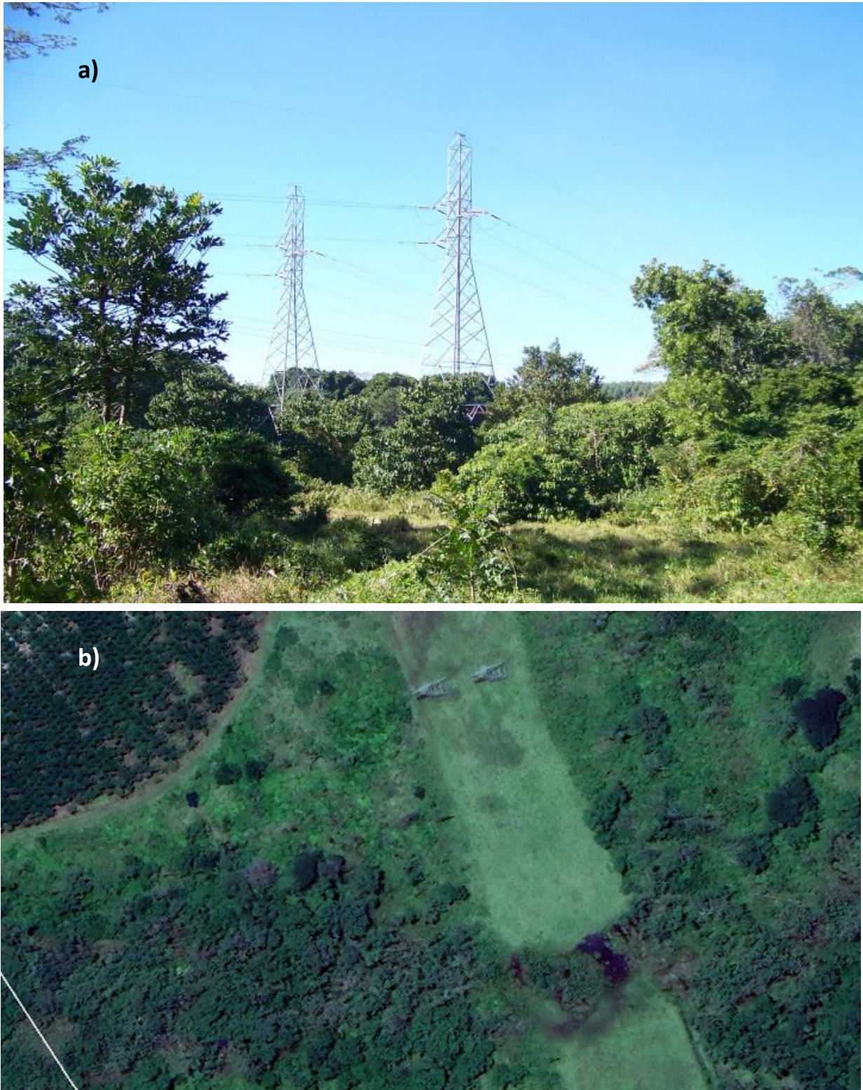
Figure 3: An example of vegetation clearance - a 132 kV line passing through a section of swamp forest vegetation in the Indian Ocean Coastal Belt biome near Port Durnford, south of Richards Bay (Photo: SDP); and B) An aerial image of the same corridor pictured in (a), indicating extent of the cleared vegetation (Google Earth, 2018).
