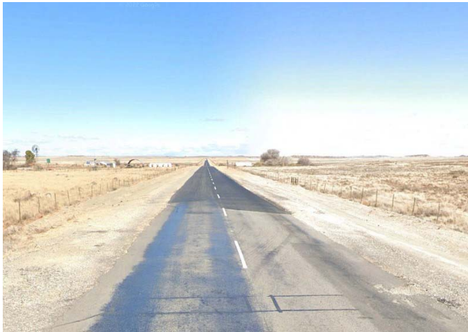
Photo 3: Southbound view along the R389
