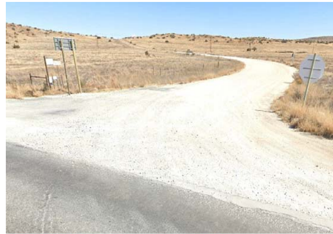
Photo 4: Westbound view Kranskop Road
