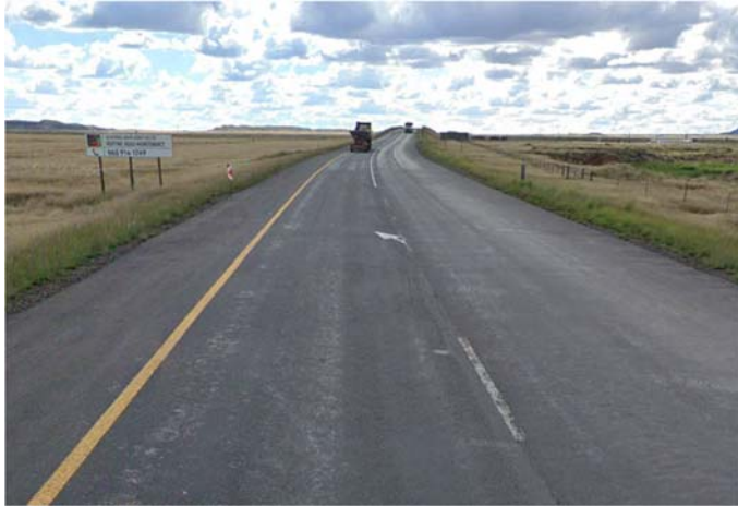
Photo 1: Northbound view along N10 towards the N1 at Hanover
