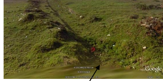
2: Downstream drainage line from Road Stormwater Culvert – crossing 2
