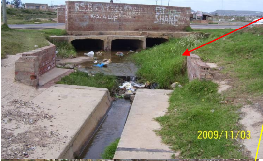
1: Culvert & Proposed pipeline crossing
