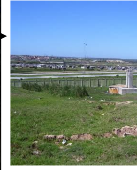
13. existing sewer vents next2 drainage line
