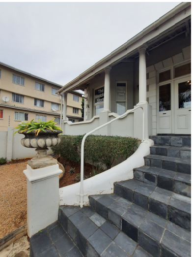
EAST ELEVATION – LOOKING SOUTH
