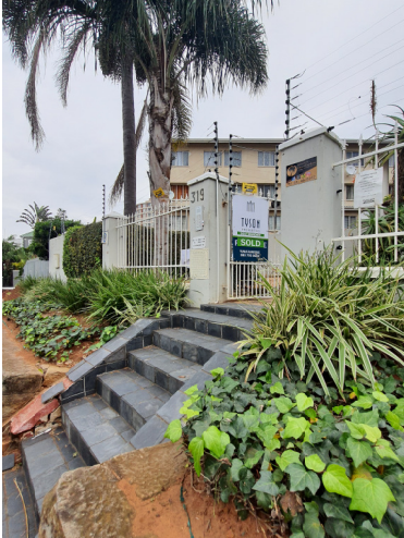
STAIRS LEADING TO ROAD
