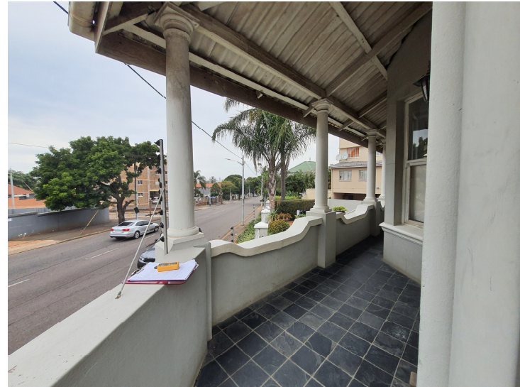
NORTH EAST CORNER OF MAIN BUILDING
