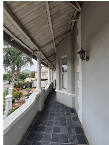
VIEW FROM PARKING DOWN EAST PORCH
