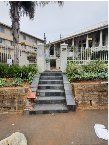
VIEW - EAST ELEVATION FROM ROAD
