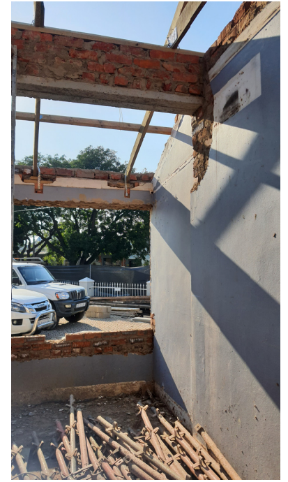
VIEW FROM INSIDE THE MEETING ROOM TOWARDS THE EAST BDRY
