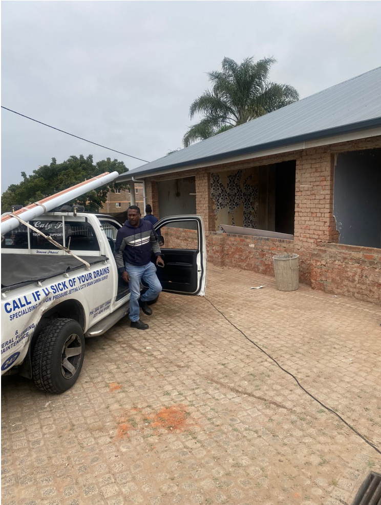
NORTH ELEVATION – UPDATED VIEW , PLASTERWORK IN PROGRESS
