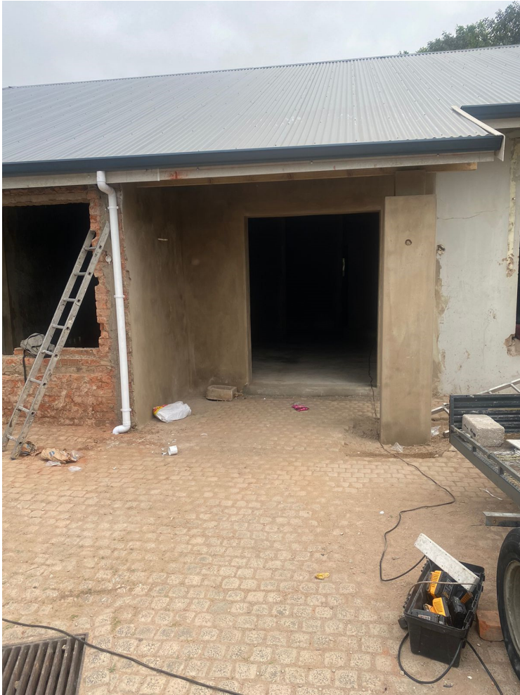
MORE UPDATED VIEW OF ENTRANCE OFF DRIVEWAY – ROOF SHEETING ADDED
