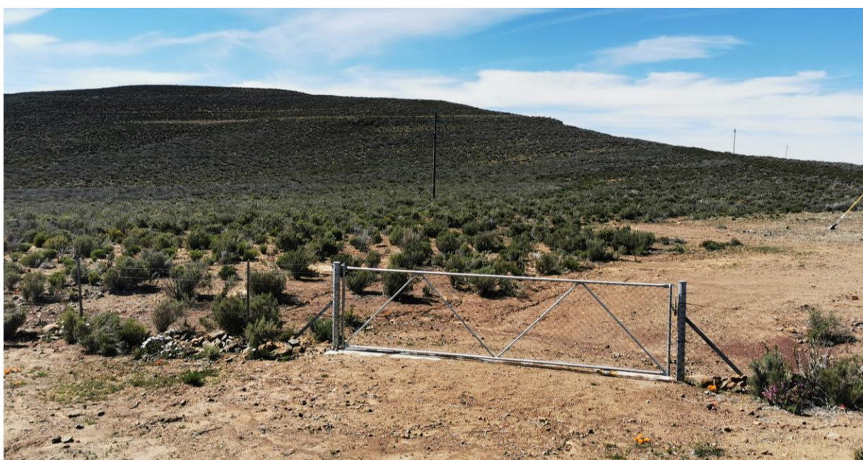
Figure 18: OHP route east of R354 road towards Komsberg substation.
