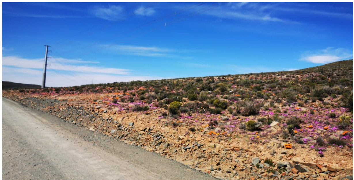
Figure 17: OHP route east of Bon Espirange substation towards R354 road.
