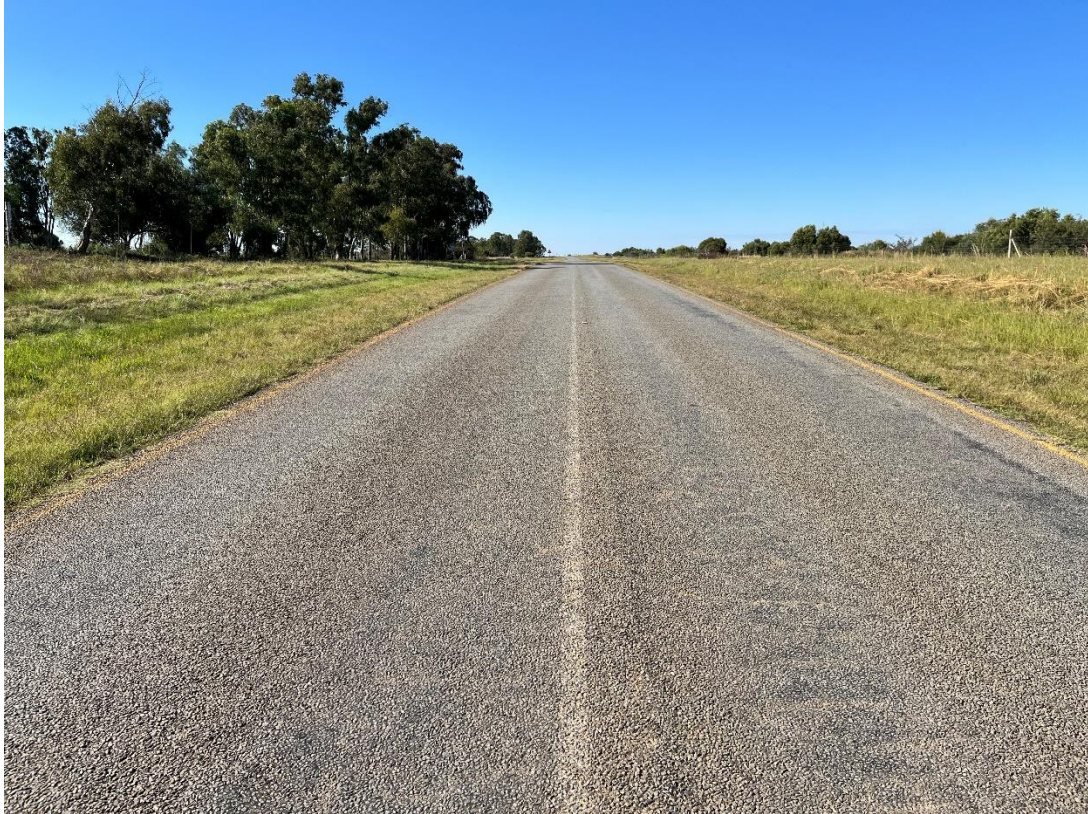
Figure 7:9 Existing Road R50505 @ Km 12.99 – South Approaching (Access 1)
