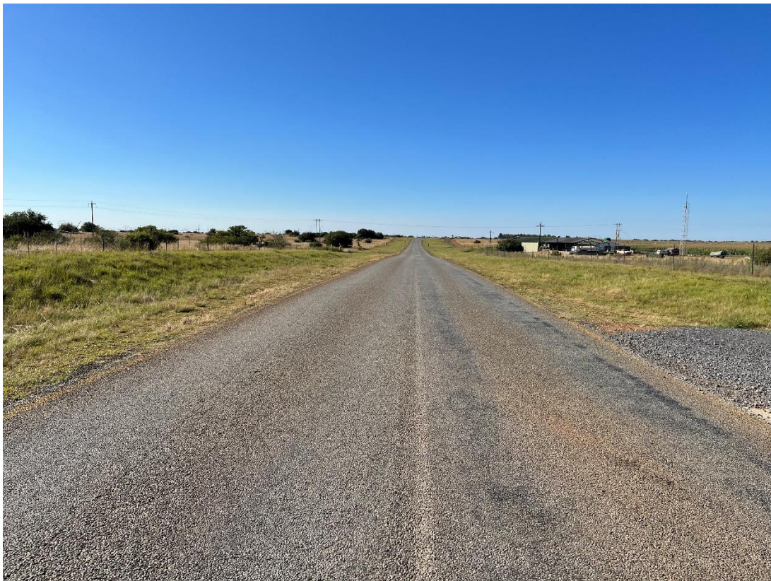
Figure 7:12 Existing Road R50505 @ Km 11.49 – South Approaching (Access 2)
