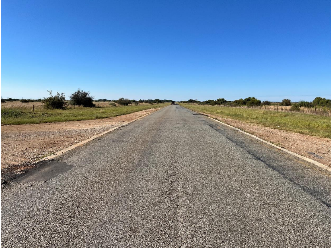
Figure 7:6 Existing Road R50505 @ Km 14.79 – South Approaching (Access 3)
