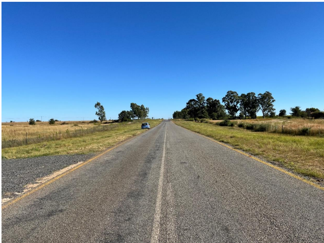
Figure 7:13 Existing Road R50505 @ Km 11.49 – North Approaching (Access 2)
