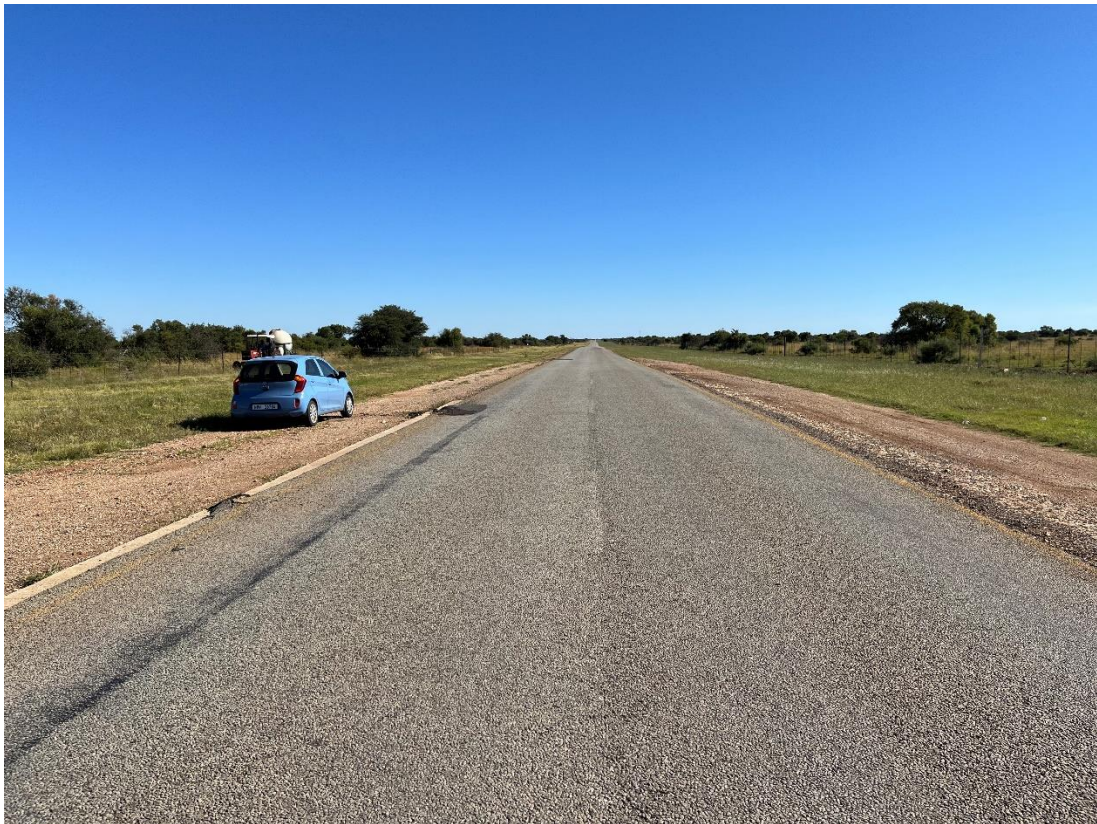
Figure 7:7 Existing Road R50505 @ Km 14.79 – North Approaching (Access 3)
