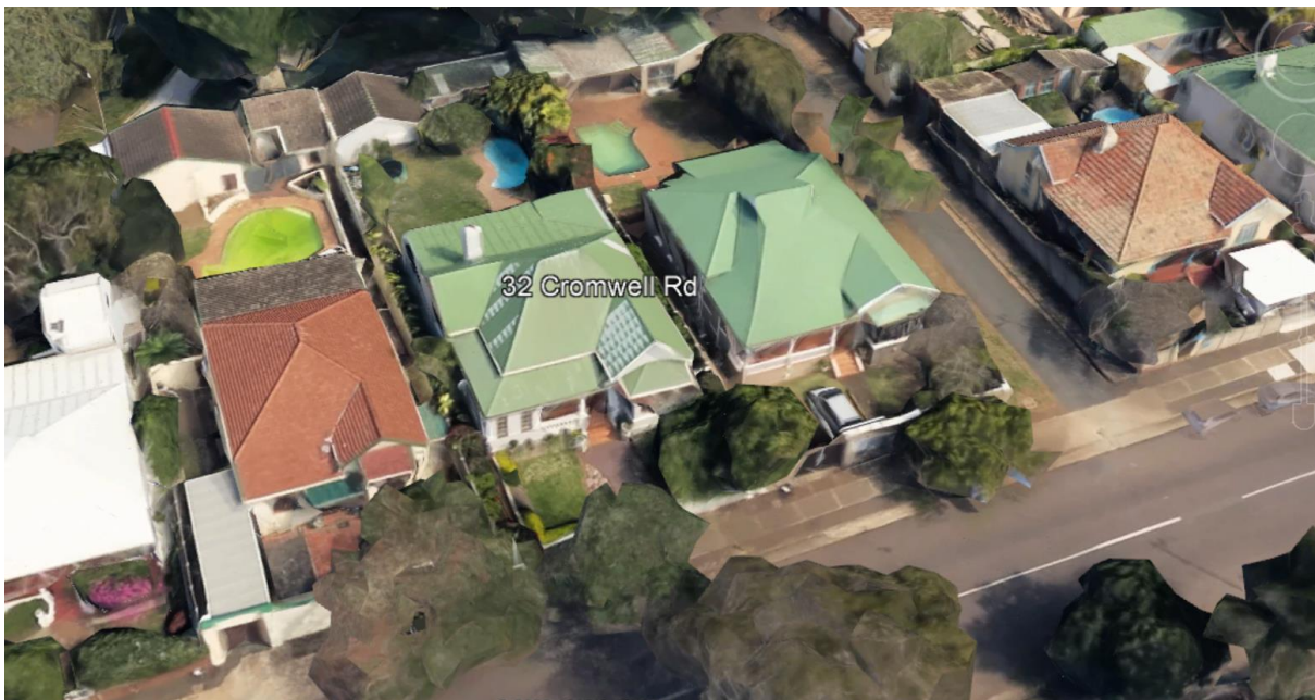
Low rise context, all buildings having asymmetrical gables and verandas.
