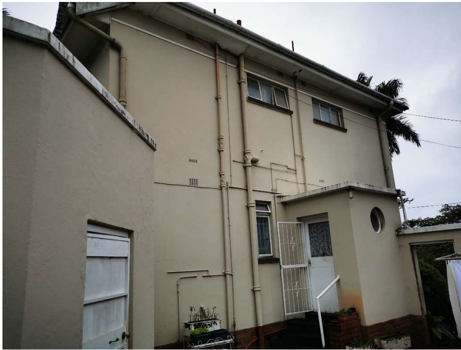
VIEW OF THE MAIN DWELLING – SIDE ELEVATION
