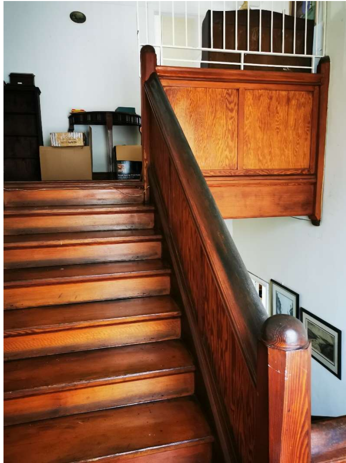
View of the Staircase – remaining unaltered
