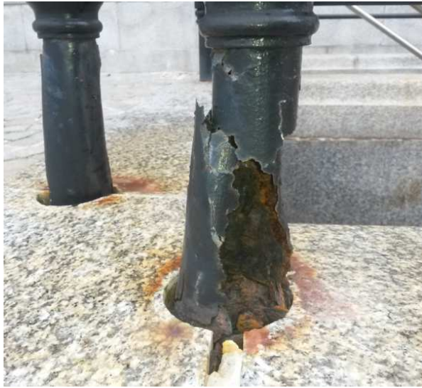
Photo 4.39 & 40: Cast Iron steelwork that is corroding should be replaced with stainless steel base fixing with sleeve and cast iron railing on top, to avoid future staining of granite.
