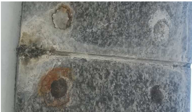
Photo 4.4 & 4.5: Skimming grout covering fixing lugs is popping off due to corrosion at the fixing lug.
