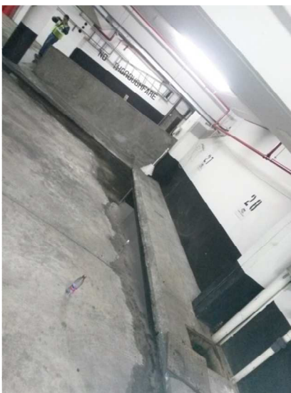
Photo 4.45 & 46: Ground water leak at bottom level of basement depositing silt from the foundations of Africa House into the basement.
