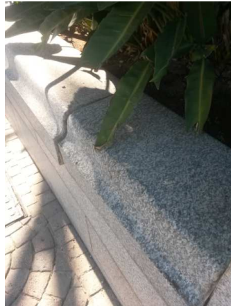
Photo 4.12-14: Lateral movement of planter box coping.
