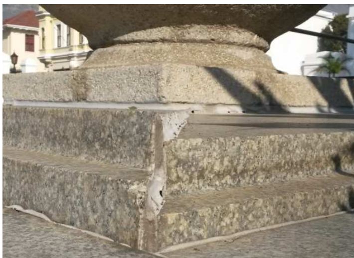
Photo 4.21: Close-up of pot plant base, where the one element has settled, while the adjoining element has not moved.
