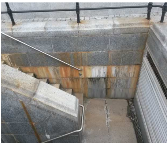
Photo 4.36-37: Abnormal efflorescence staining – possibly a block underground drain & also corrosive staining
