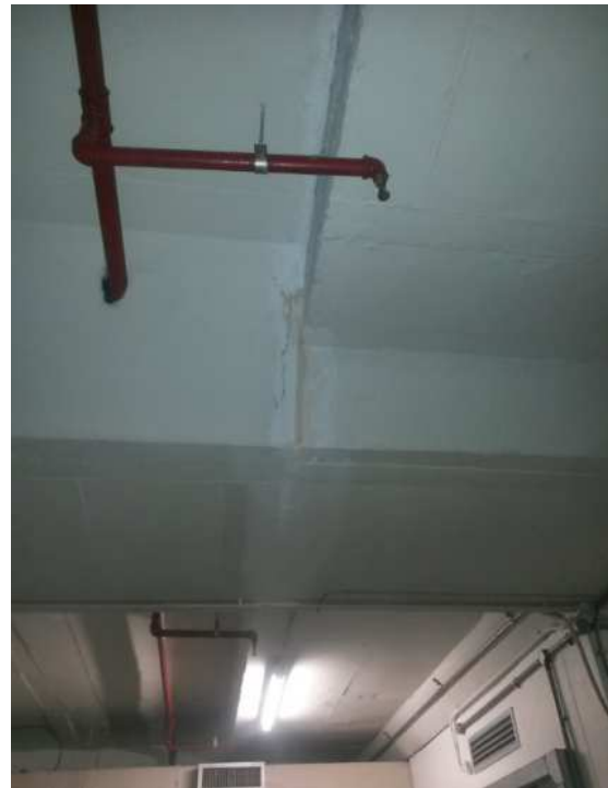
Photo 4.43 & 44: Movement joint +/- 40m from basement entrance, to be made good and waterproofing on top of slab to be reviewed on site.
