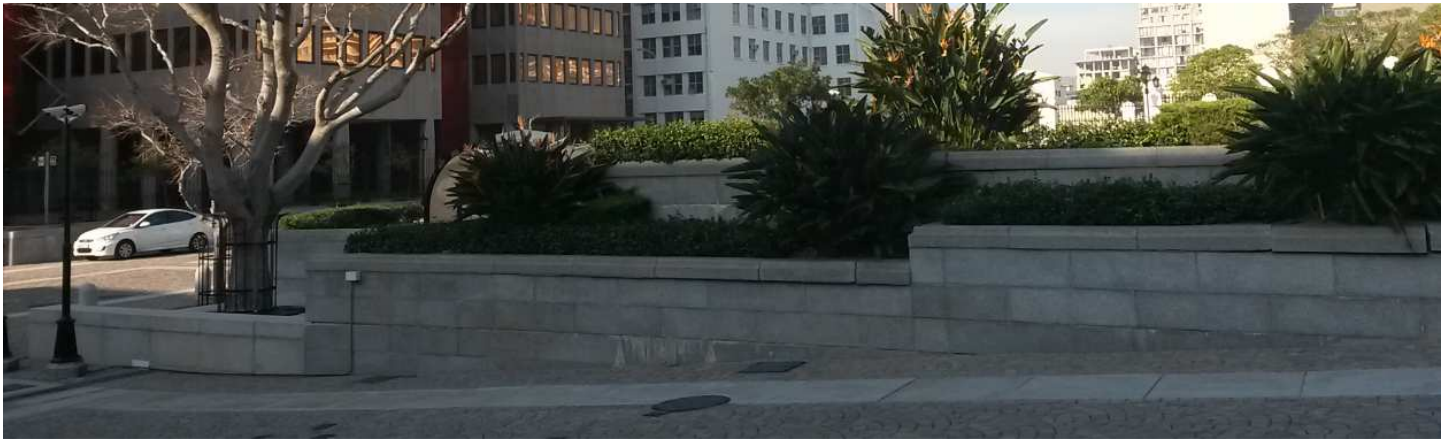
Photo 4.11: Granite planter boxes with lateral movement of coping and vertical movement of cladding elements & efflorescence visible
