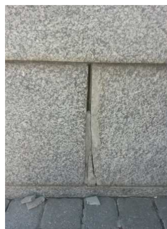
Photo 4.8-10: Granite elements on top of curved entrance where movement of elements have occurred.
