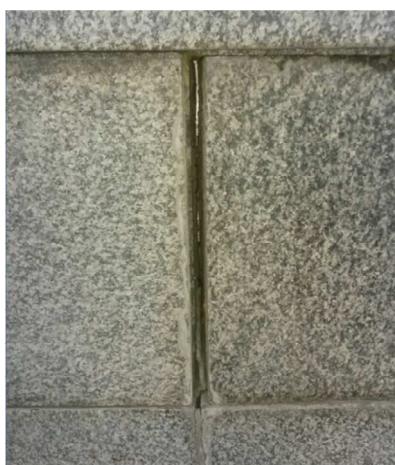
Photo 4.8-10: Granite elements on top of curved entrance where movement of elements have occurred.
