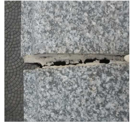
Photo 4.11: Granite planter boxes with lateral movement of coping and vertical movement of cladding elements & efflorescence visible
