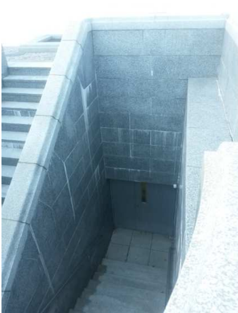
Photo 4.34-35: Typical efflorescence staining from rainwater running down granite facade
