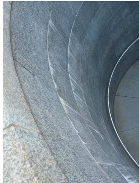
Photo 4.34-35: Typical efflorescence staining from rainwater running down granite facade
