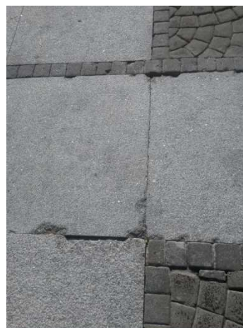
Photo 4.24 & 25: Granite slabs with exposed joints & chipped edges
