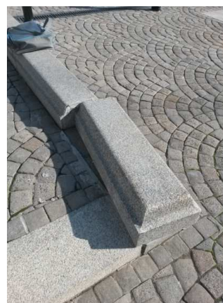
Photo 4.26 & 27: Standing water underneath granite slabs at basement emergency exit and granite kerb that has been dislodged.
