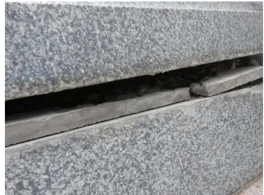
Photo 4.15-16: Vertical movement of planter box cladding elements
