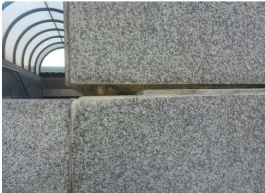
Photo 4.15-16: Vertical movement of planter box cladding elements
