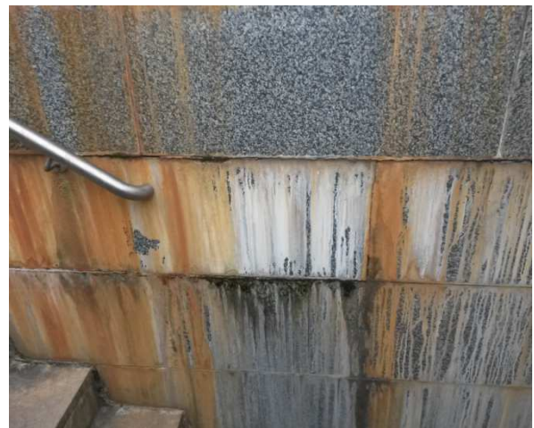
Photo 4.36-37: Abnormal efflorescence staining – possibly a block underground drain & also corrosive staining
