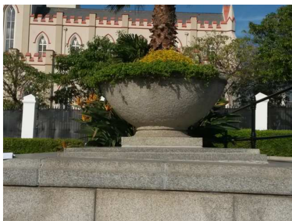
Photo 4.18-19: Plinths with visible differential settlement of +/- 20mm on a number of plinths at the potplant base.
