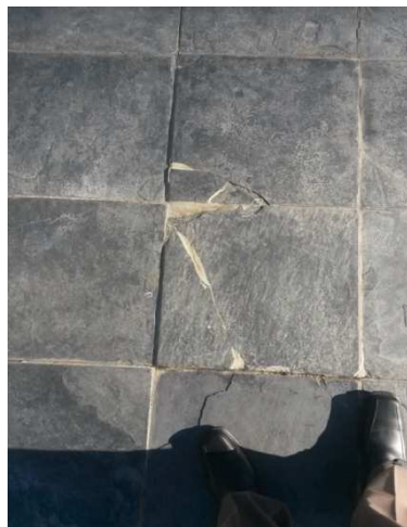
Photo 4.31-33: Cracked and damaged slate tiles.
