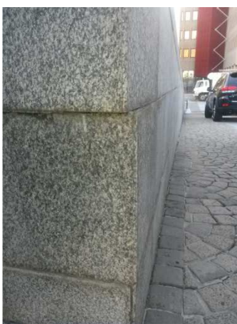
Photo 4.8-10: Granite elements on top of curved entrance where movement of elements have occurred.
