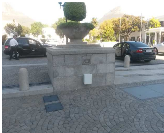
Photo 4.18-19: Plinths with visible differential settlement of +/- 20mm on a number of plinths at the potplant base.
