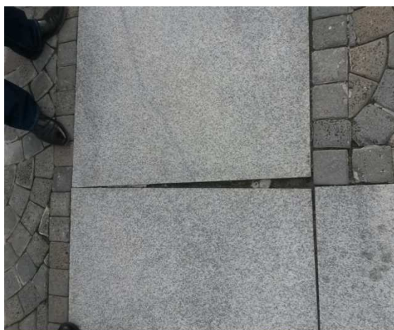
Photo 4.24 & 25: Granite slabs with exposed joints & chipped edges
