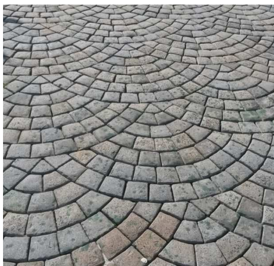
Photo 4.30: Paving cobbles that are in need of treatment to remove paint marks
