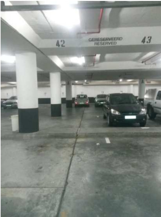
Photo 4.43 & 44: Movement joint +/- 40m from basement entrance, to be made good and waterproofing on top of slab to be reviewed on site.
