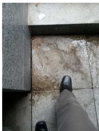
Photo 4.26 & 27: Standing water underneath granite slabs at basement emergency exit and granite kerb that has been dislodged.
