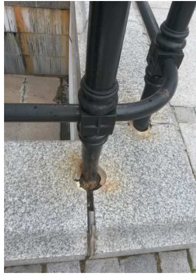
Photo 4.39 & 40: Cast Iron steelwork that is corroding should be replaced with stainless steel base fixing with sleeve and cast iron railing on top, to avoid future staining of granite.
