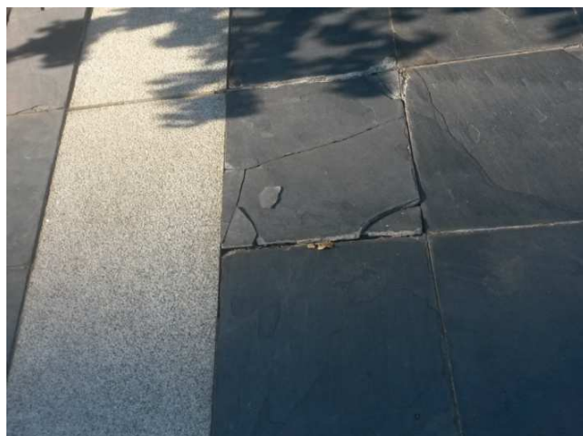
Photo 4.31-33: Cracked and damaged slate tiles.
