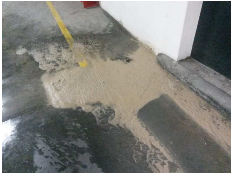
Photo 4.45 & 46: Ground water leak at bottom level of basement depositing silt from the foundations of Africa House into the basement.
