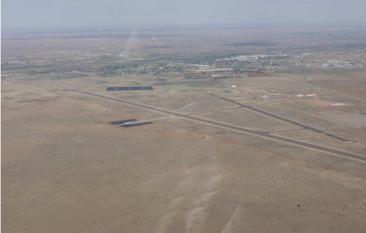
Plate 17, Existing solar arrays at Upington Airport as seen from the air
