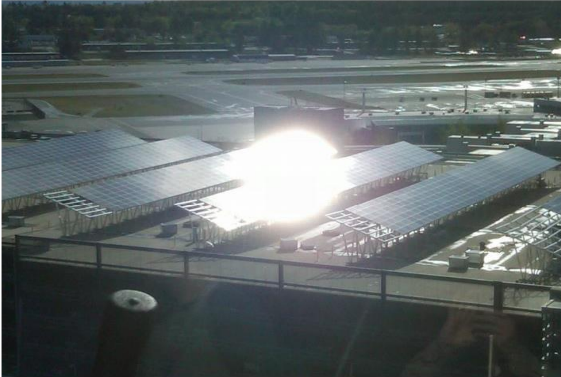
Plate 21 - Glare experienced in the Control Tower at Boston Regional Airport from an adjacent PV array
