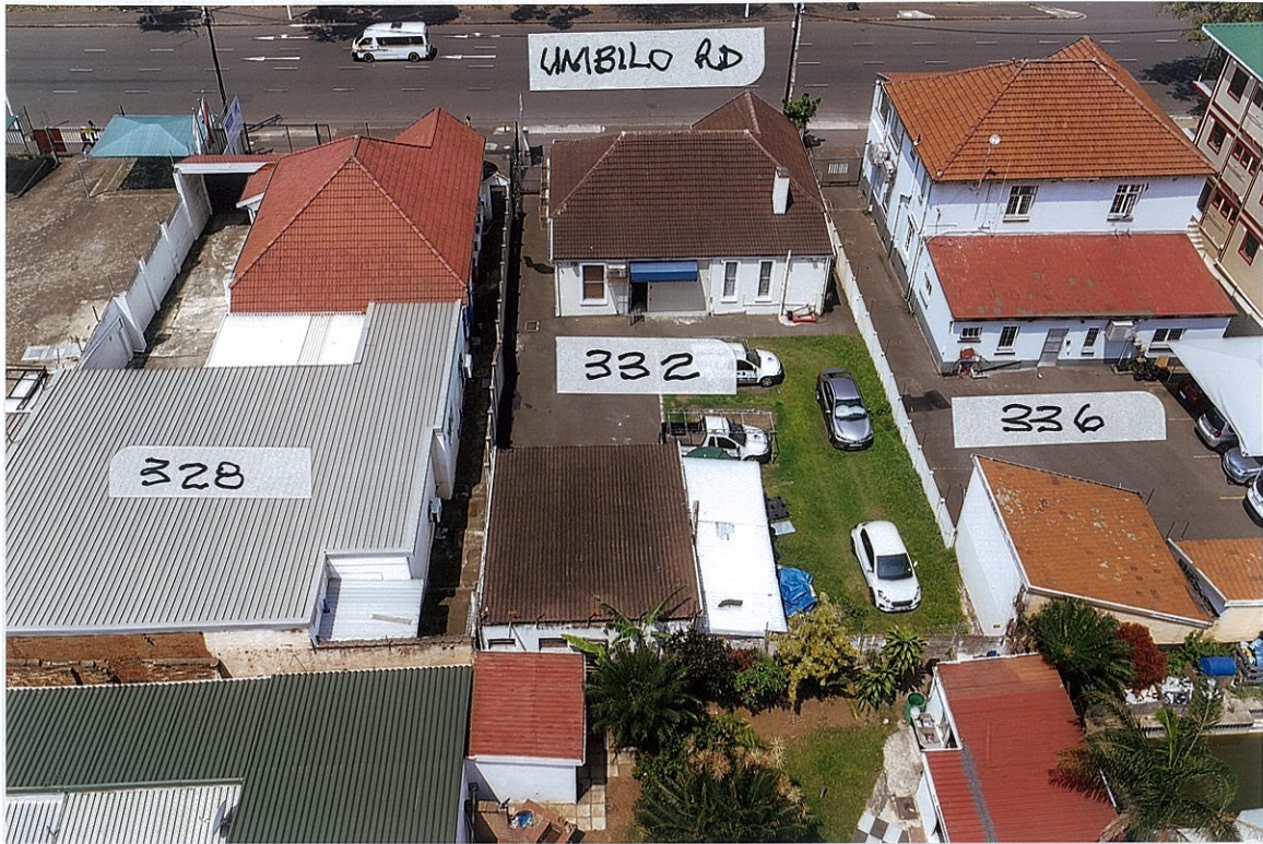
AERIAL VIEW TAKEN FROM REAR OF THE PROPERTY & ADJACENT PROPERTIES.
