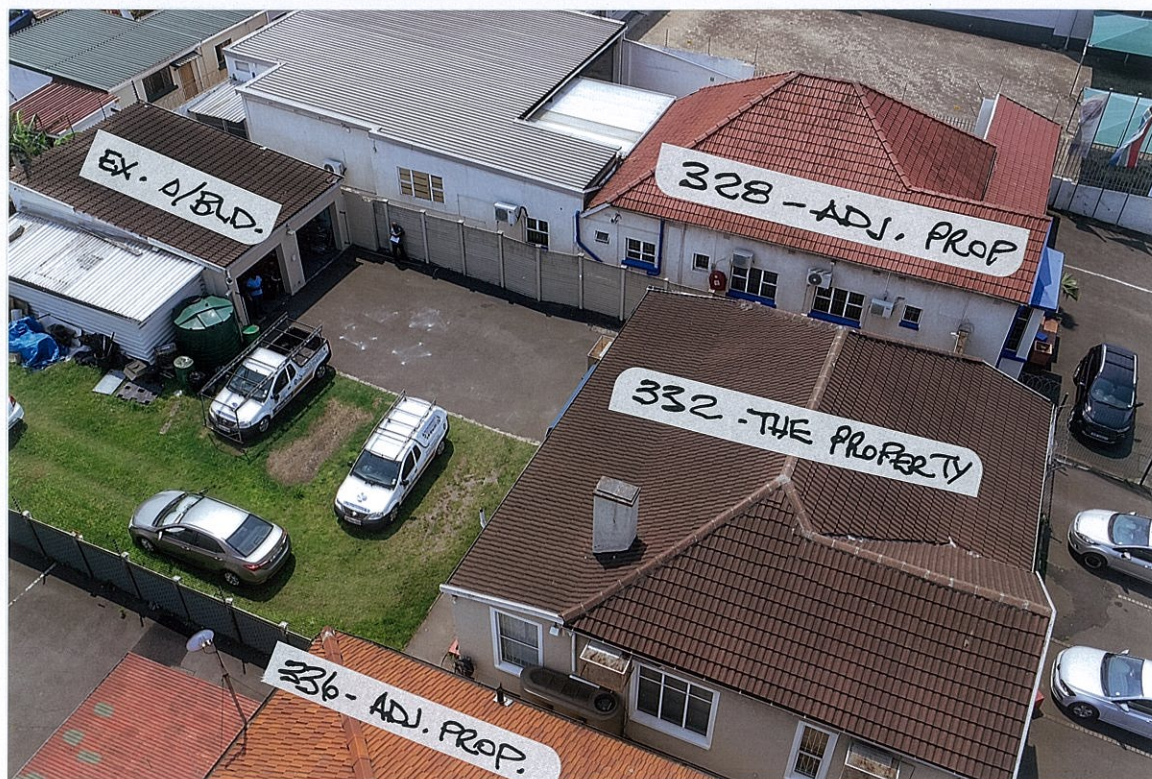
SIDE VIEW OF ADJ. PROPERTY 328 UMBILO RD + THE PROPERTY IN THE FOREGROUND.
