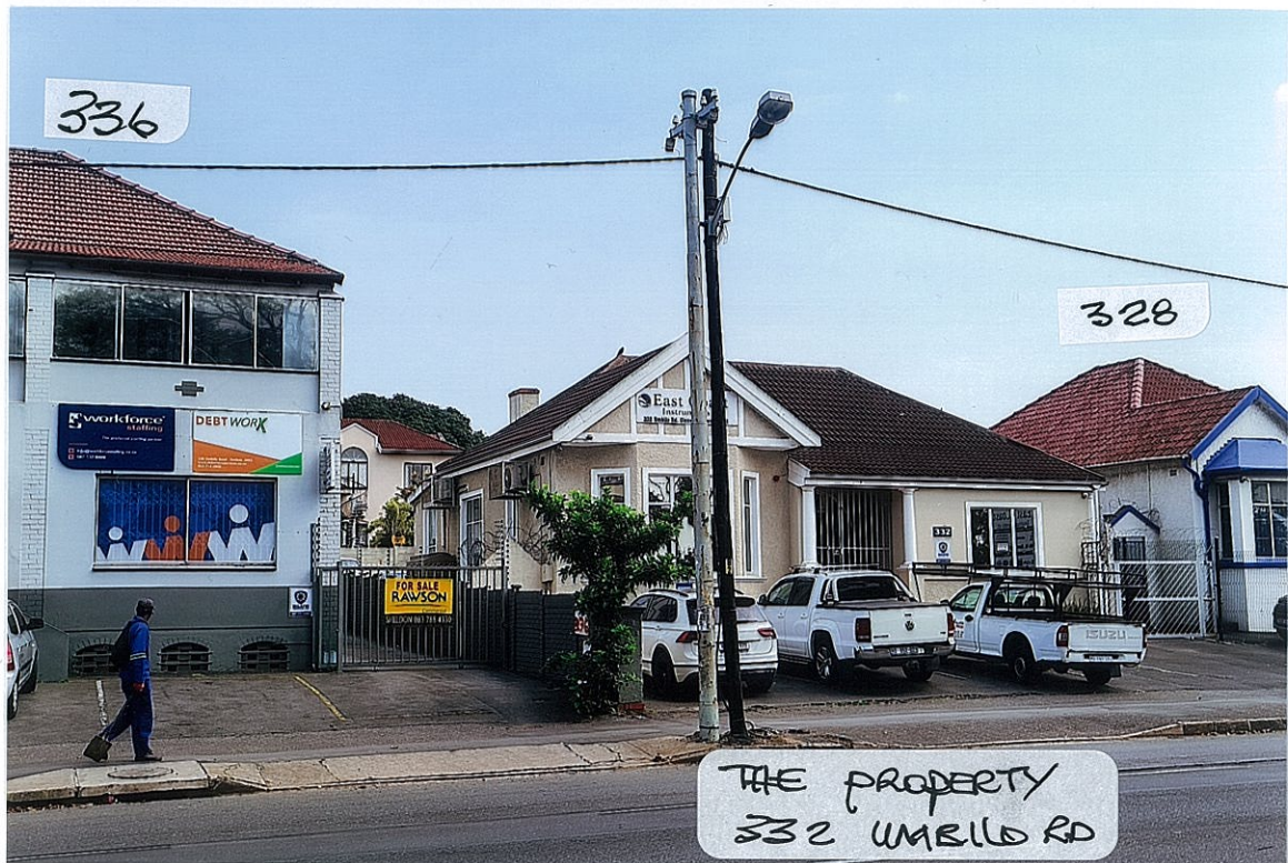
332 UMBILO RD - EAST COAST INSTRUMENTS SIDE & STREET FRONTAGE VIEW. ADJ. PROPERTIES TO THE LEFT & RIGHT.
