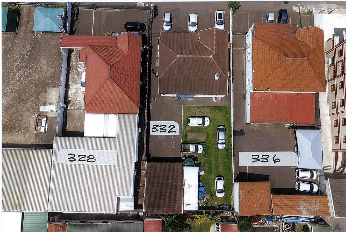
AERIAL VIEW TAKE DIRECTLY ABOVE 332 UMBILO RD + ADJ. PROPERTIES.
