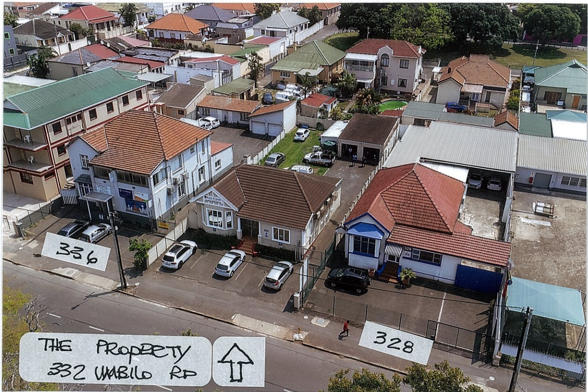
UMBILO RD AERIAL VIEW WITH ADJACENT PROPERTIES
