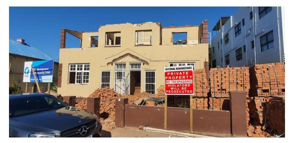
The existing building is a double story building with brick and mortar walls and a concrete slabs.
