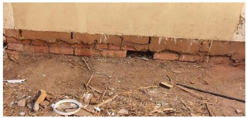
As the demolition of the internal brickwork on the first floor continues there is a risk of the further movement and damage to the external brickwork. This will result in the external brickwork on the first floor being unstable and unsafe, which poses a huge threat to the workers on site as well as the neighbouring properties.
