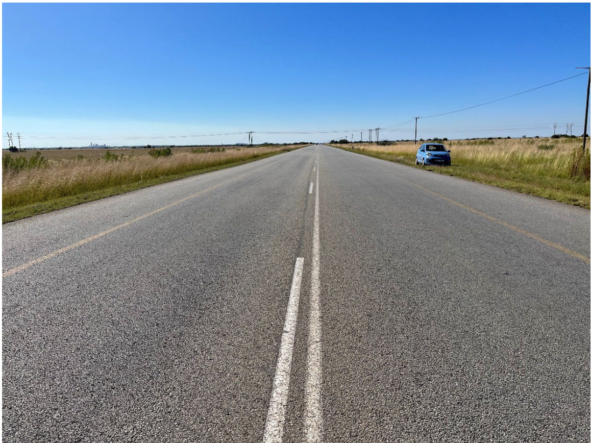
Figure 7.6 Existing Road P28-4 @ Km 7.15 – East Approaching (Access 1)
