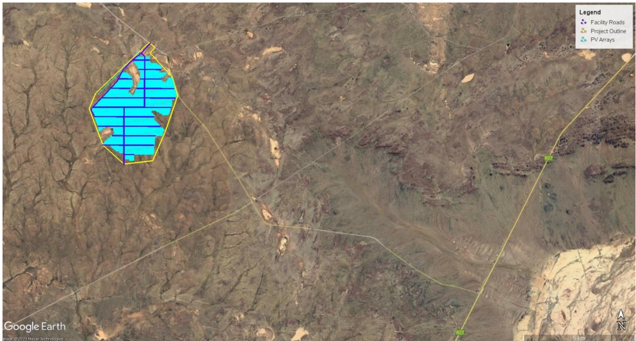
Figure 1. Satellite image showing the location of the proposed Kotulo Tstatsi PV 3 development, west of the R27, located between Kenhardt and Brandvlei.
