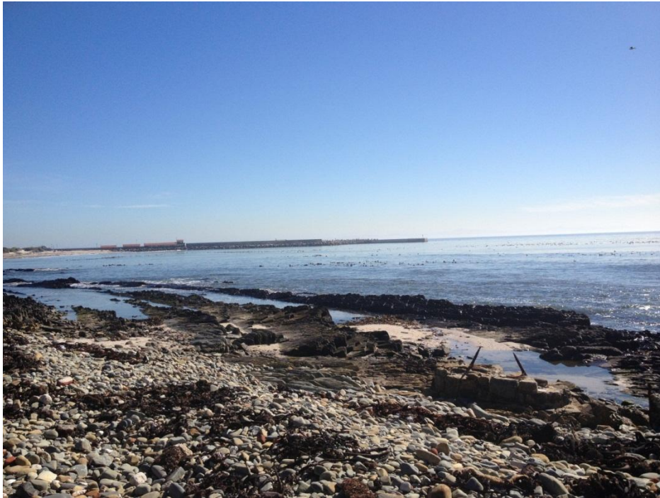
Figure 3. Looking north towards Murray's Beach and the harbour from the location of the existing sewer outfall
