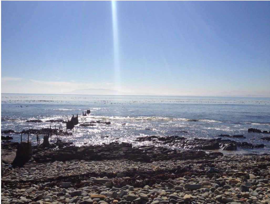
Figure 5. Looking out to sea, northeast, along the existing sewer outfall. [Visible structures are supports from demolished pipe lines]
