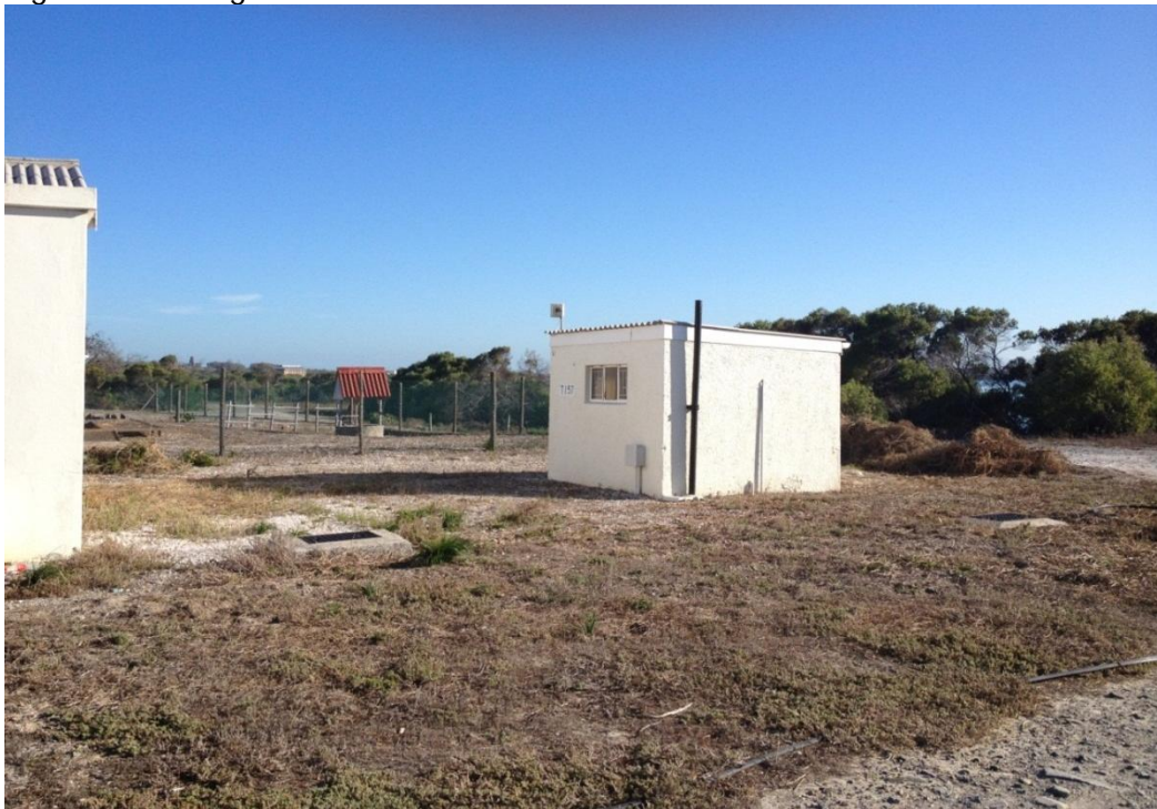
Figure 10. Looking northwest from the location of the proposed SPP at the dog unit complex
