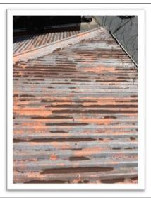
Some roofs are laid at a 2° slope, which is too shallow an angle to provide sufficient run-off during bouts of rain.
