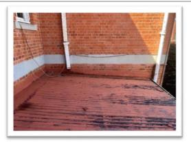
The valleys on some of these sheet metal roofs were incorrectly waterproofed, in a possible attempt to counter the leaks. These roofs will leak because of the shallow slope, allowing water ingress to the areas below.
