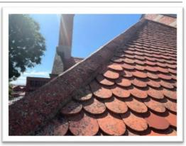
Water ingress onto ceilings and down walls are also results of dislodged and broken tiles. It was noted that the underlay, which acts as a waterproof barrier under the tiles, was also damaged in several places across the footprint of the building, which would allow water to penetrate onto ceilings and the timber trusses.
