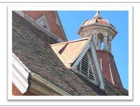
In general, these require all the flashing joints and ridges to be re-formed to seal and join together properly. Paint has weathered significantly and is peeling off these sheets and joints.
