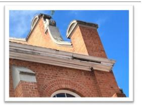
In other instances, the roof overhangs are not sufficient enough to discharge water into the gutter, which would result in water ingress into the building.
