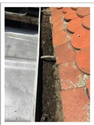
Structural failure of a number of these gutters can be attributed to the failure of the timber fascia they are fixed to, where the fascia have rotted or pulled away from their support structure.
