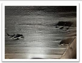
In roof valleys, it was evident that in several areas, the overlap joint between the metal valley and tile-edge was compromised, due to movement of the tiles. In several instances, the resulting leaks were poorly waterproofed with a waterproof membrane and bitumen paint, which is considered a temporary solution.
