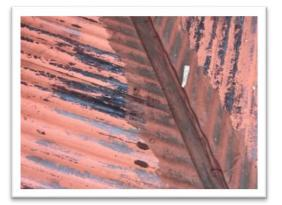
Loose fixing of some roofs was also noted, which may also indicate failure of the timber battens below because of old age and/ or rot.
