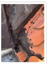
Flashing and counter flash waterproofing, where the tiles meet brickwork, is in most cases either missing, not correctly installed or poorly installed.
