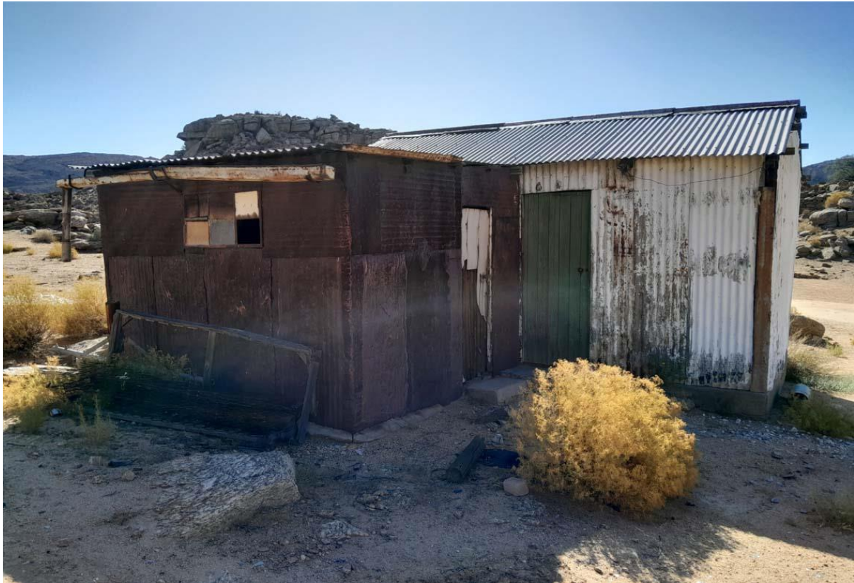
Photo E.5: NSR10 location (noise sensitive)
