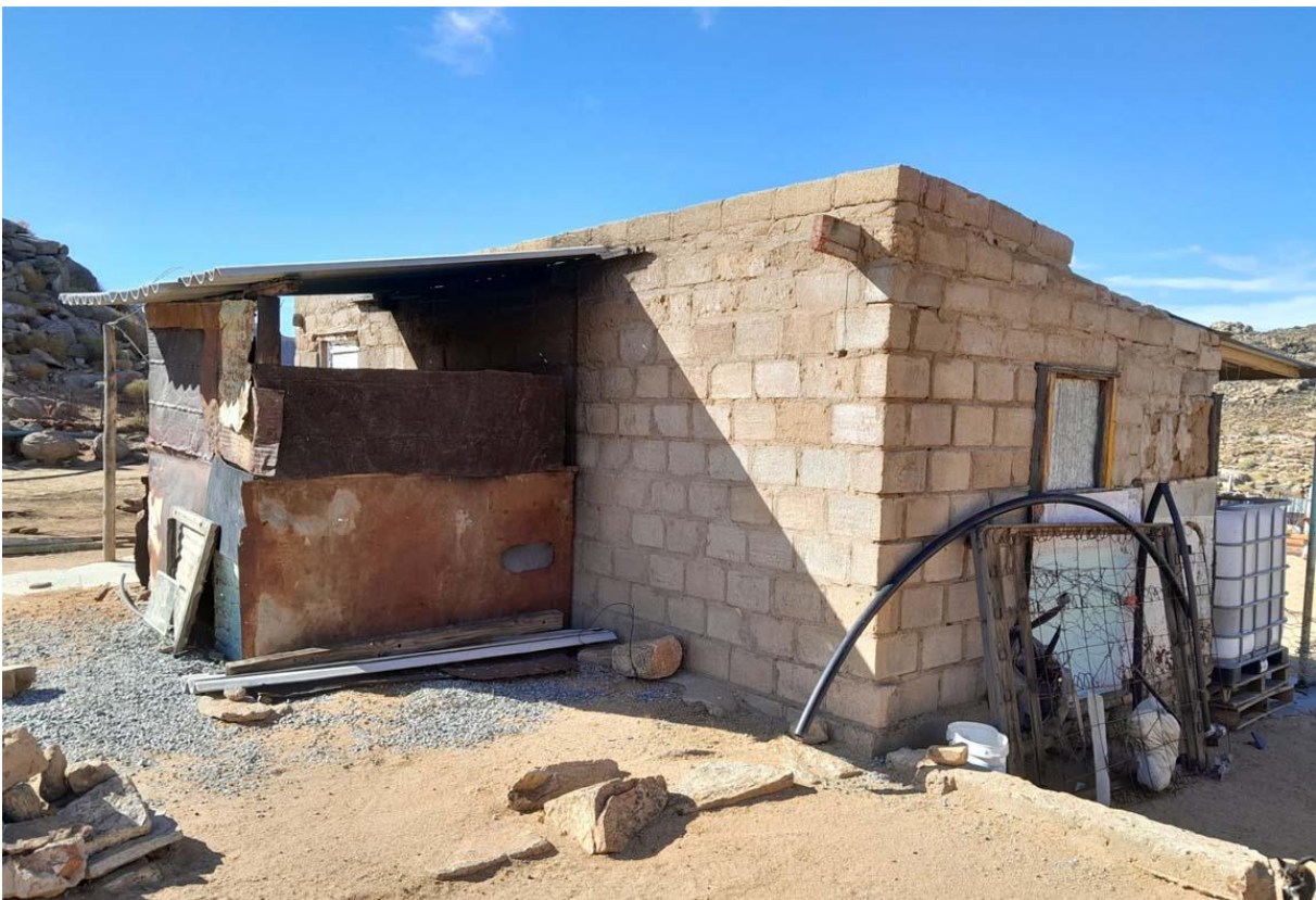
Photo E.4: NSR9 location (noise sensitive)
