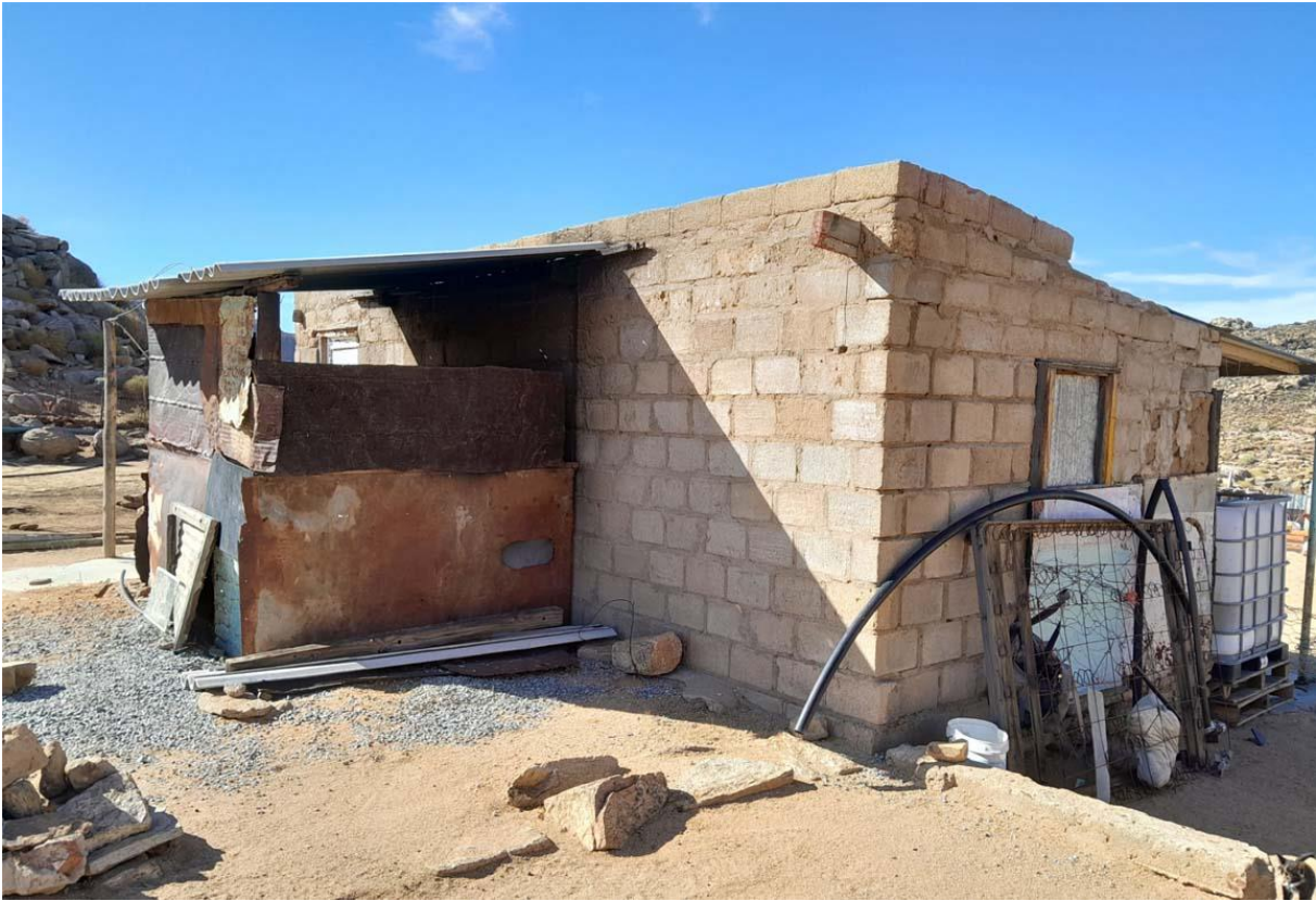
Photo E.3: NSR8 location (noise sensitive)
