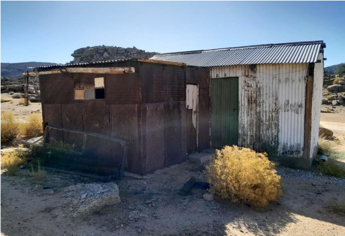
Photo E.5: NSR10 location (noise sensitive)
