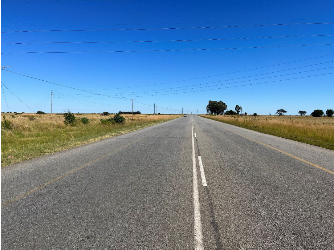
Figure 7.7 Existing Road P28-4 @ Km 7.15 – West Approaching (Access 1)
