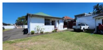
MAIN BUILDING NORTH EAST ELEVATION
