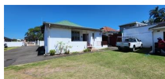
MAIN BUILDING NORTH EAST ELEVATION
