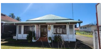
MAIN BUILDING SOUTH WEST ELEVATION
