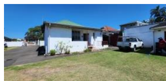
MAIN BUILDING NORTH EAST ELEVATION
