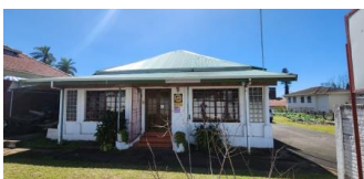
MAIN BUILDING SOUTH WEST ELEVATION
