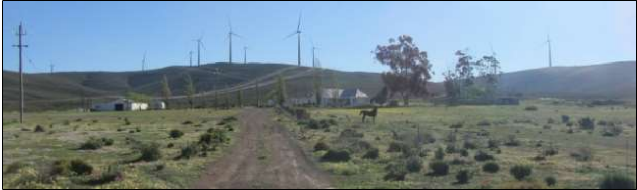
Photograph 3.7: Farmstead and outbuildings on Bona Esperance seen from entrance road. Note the turbines (Roggeveld WEF) and overhead lines feeding into Bon Espirange substation. The impact is contained to the west and south of the farmstead
