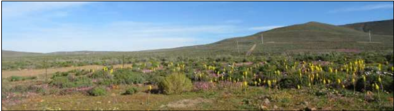
Photograph 3.12: Newly constructed line from the Roggeveld WEF to Eskom Komsberg, seen from access road to Bona Esperance
