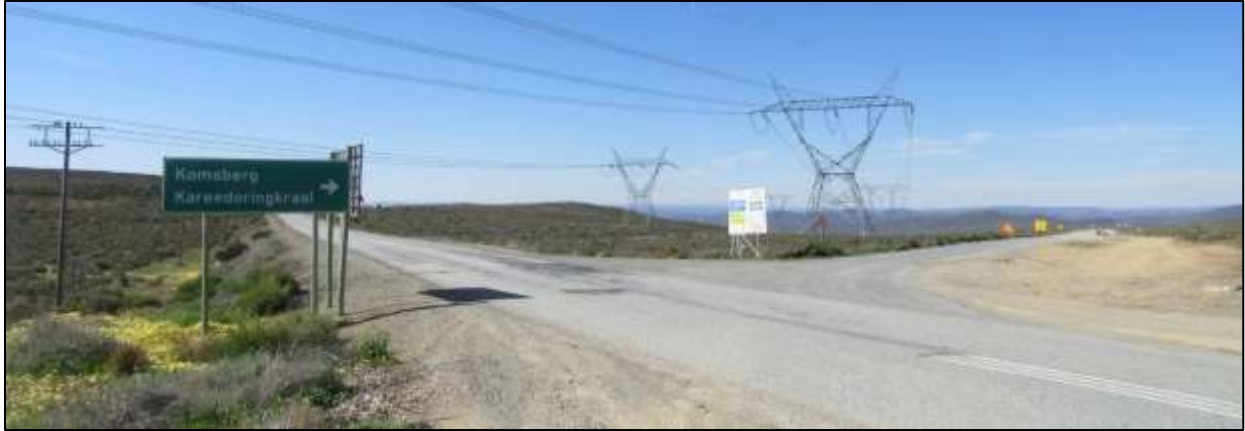
Photograph 3.1: R354-Komsberg road intersection and 756 kV and 400 kV lines viewed from the south.
