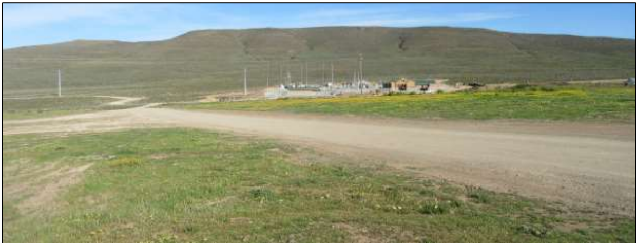
Photograph 3.10: Roggeveld WEF substation on Bona Esperance viewed from near the farmstead located to the north-west
