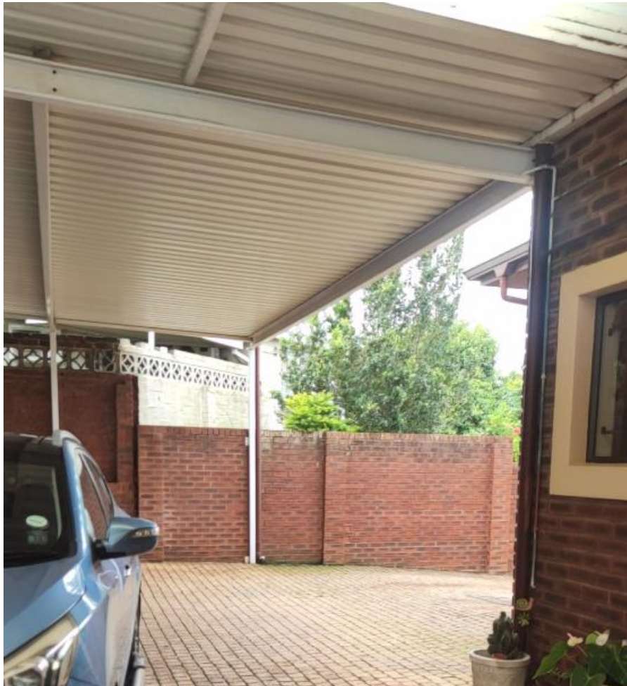
Figure 10. Image illustrates the existing awning over the garage entrance extending to the kitchen that is to be altered according to the attached plans
