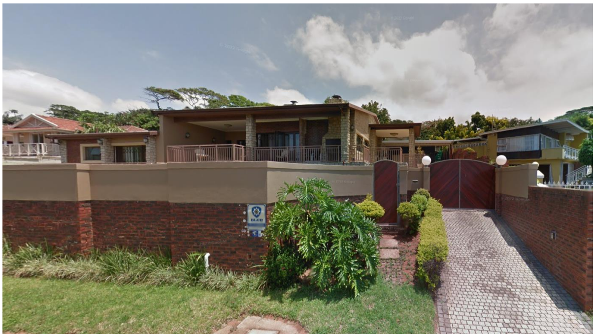
A2. Image illustrates the Baines Road facing boundary wall
