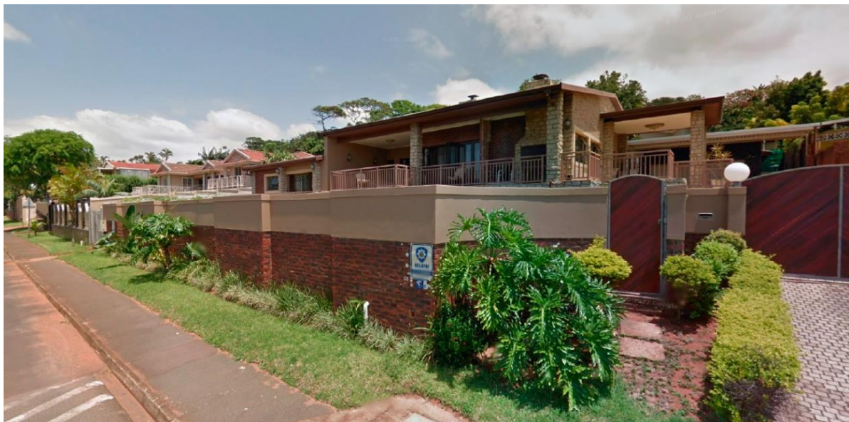
Figure 3 Image of street elevation on Baines Road which depicts exposed face brick and plaster brick boundary wall
