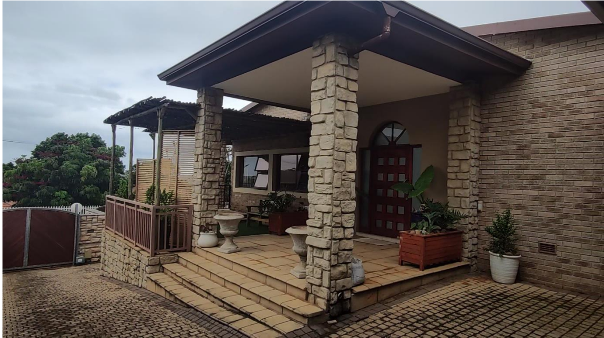
Figure 4 Image of the South Eastern Elevation of the property. Façade and columns of face brick with the existing pergola .
