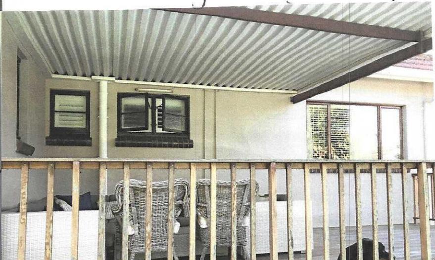
Awning - S.E. Elevation ↓
