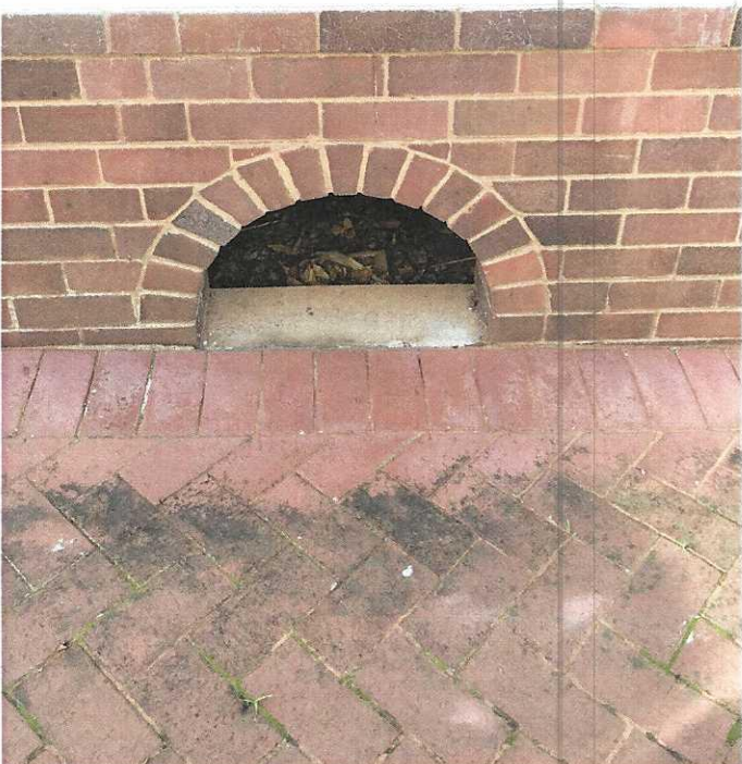
Brick detail - Air ventilation
