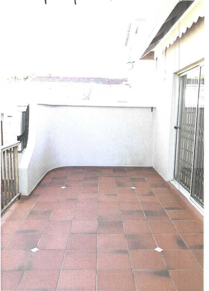
Existing open verandah - S.E.
