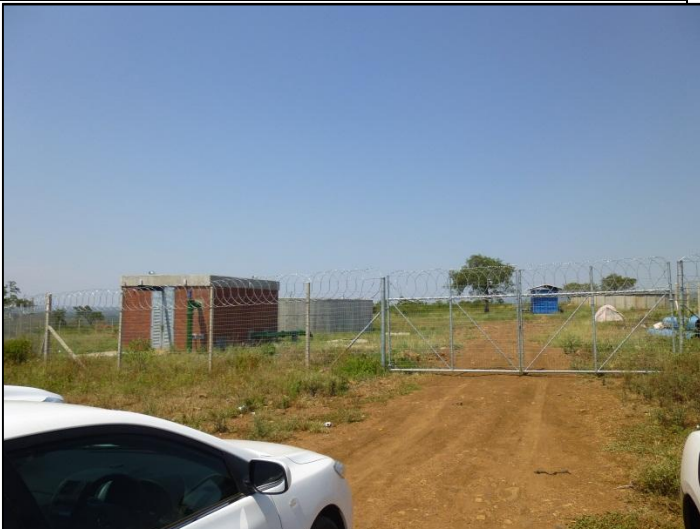
Figure B2 Existing KwaNdlazi Reservoir
