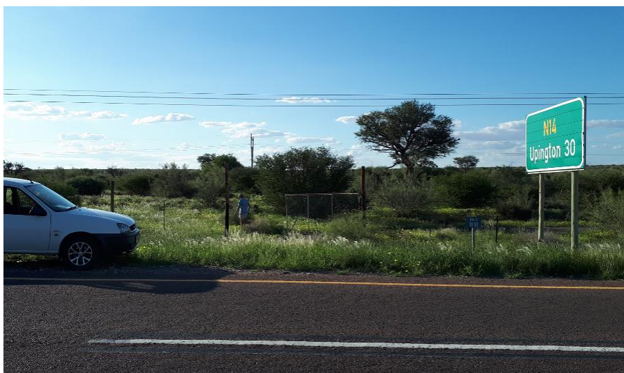
Figure 3-10: Existing Access Point 2
