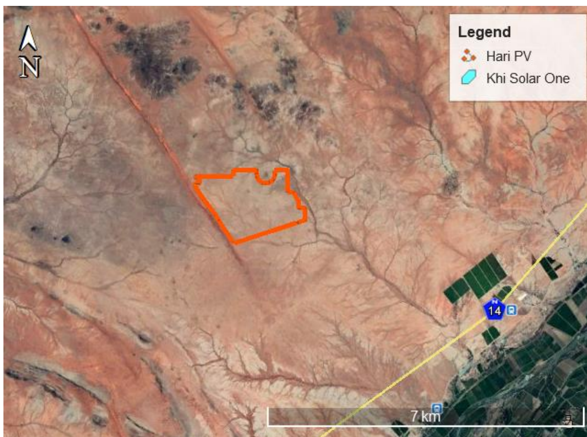
Figure 3-1: Aerial View of Proposed Hari PV Development
