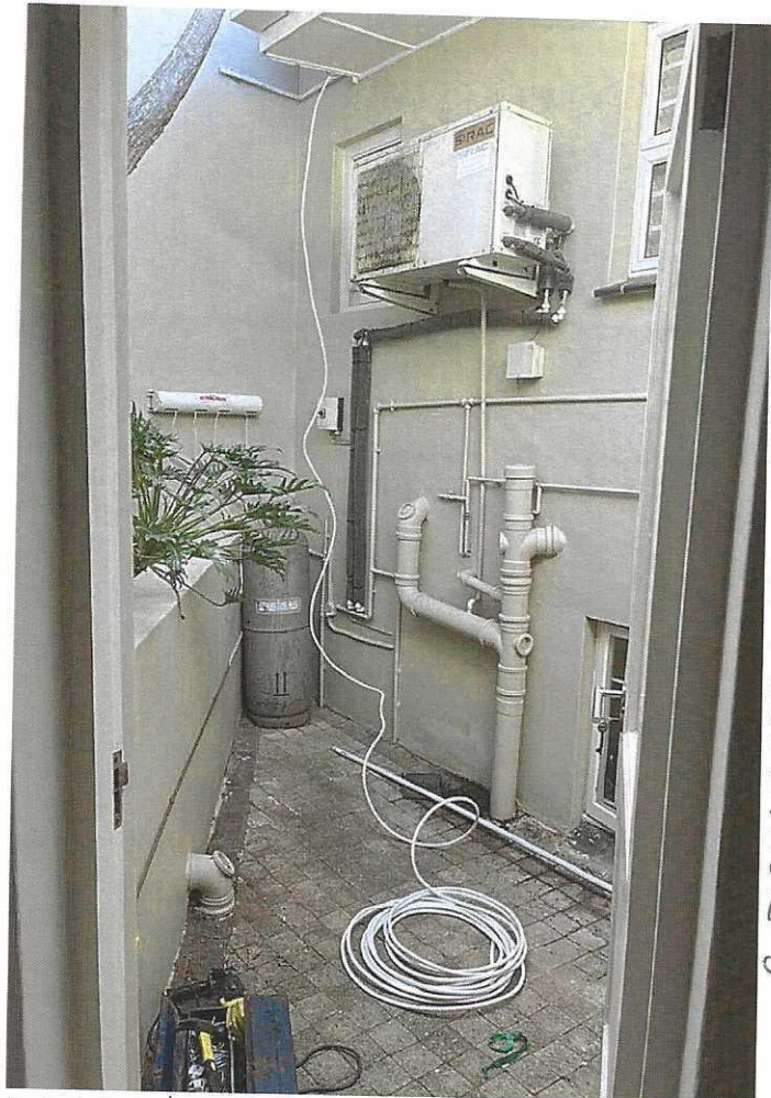
View into open yard from new staircase
