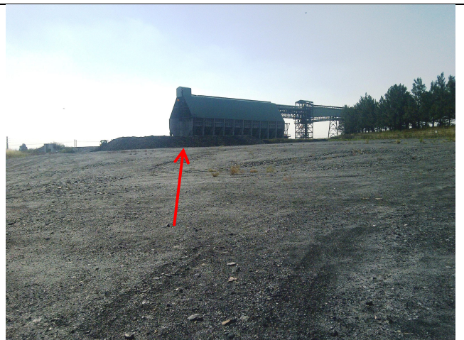
l) Syferfontein bunker storage before transfer to Sasol overland conveyor
