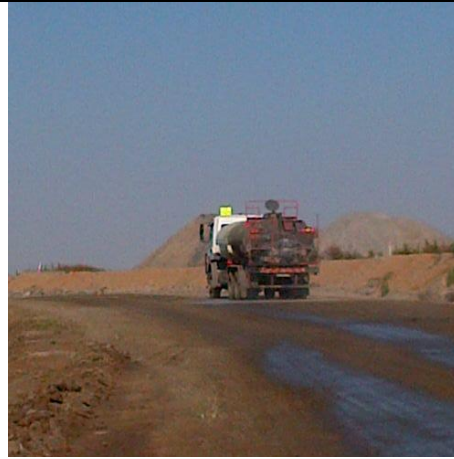
h) Dust suppression along haul and access roads
