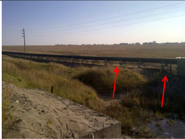
a) Overland conveyor covered with metal sheeting
