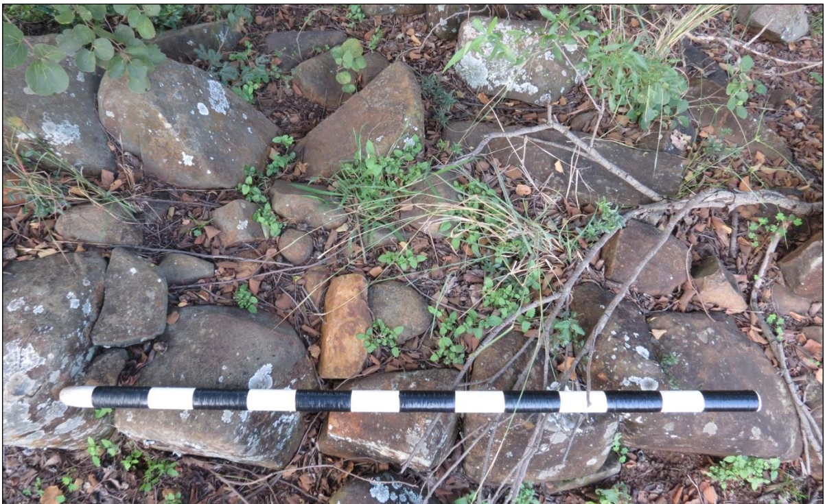
Figure 129 – Cross-view of a section of the straight walls enclosing two sides of the site. Scale in 10cm increments. Note the use of large rocks on the outside with smaller rocks in-between.
