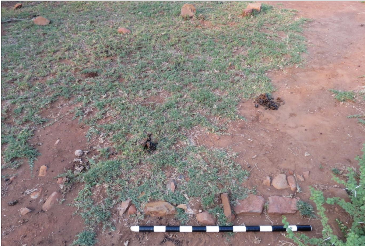
Figure 130 – A section of the foundation of the rectangular structure can be seen in the foreground. Scale in 10cm increments.
