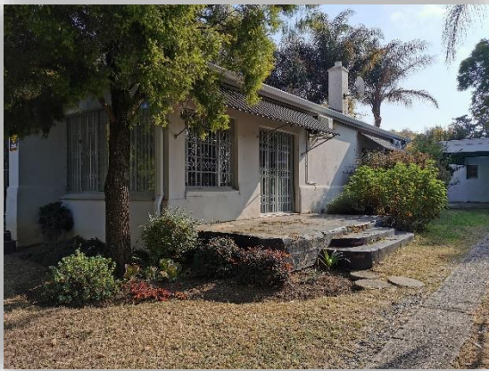
Side View of House – Side Main Veranda
