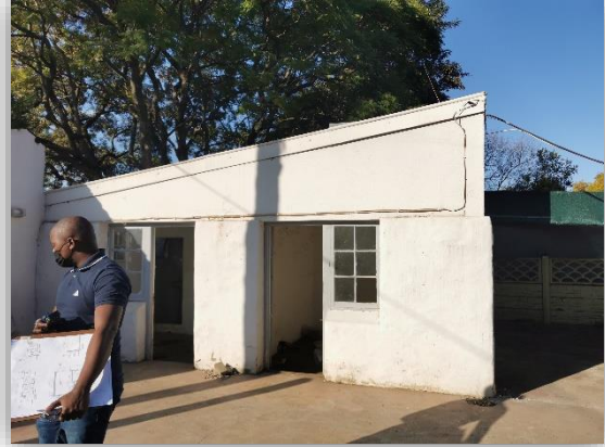
Side View of Outbuilding
