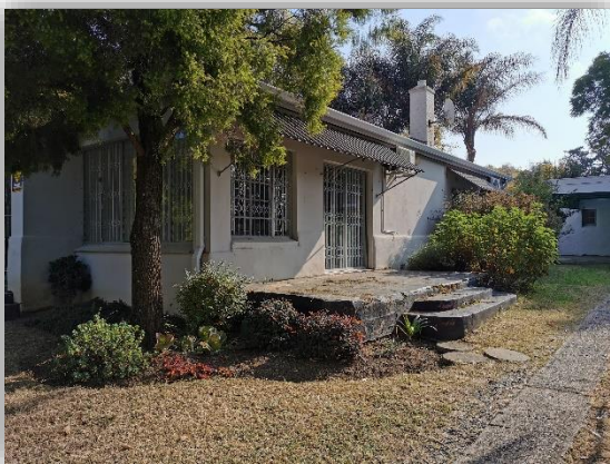
Side View of House – Side Main Veranda
