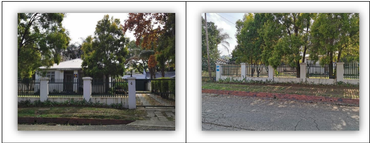
Picture – View from Street (4 White Road)
