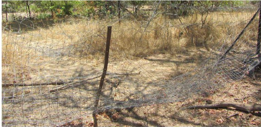
Fence damaged by the crossing of elephants.
