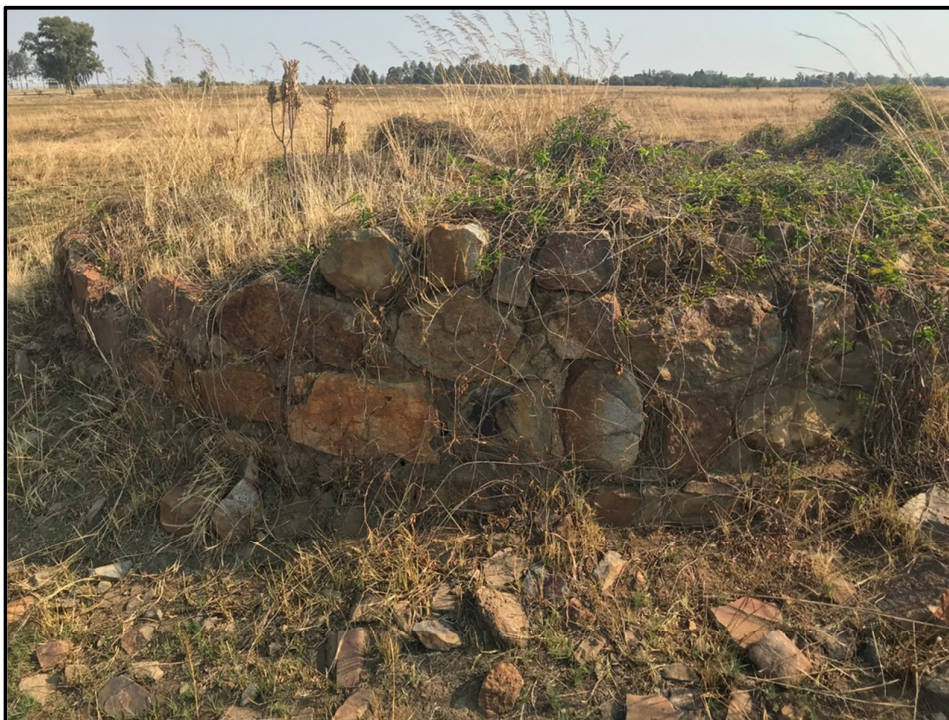
Photo 6: Old broken down structure in the southern area of the study site
