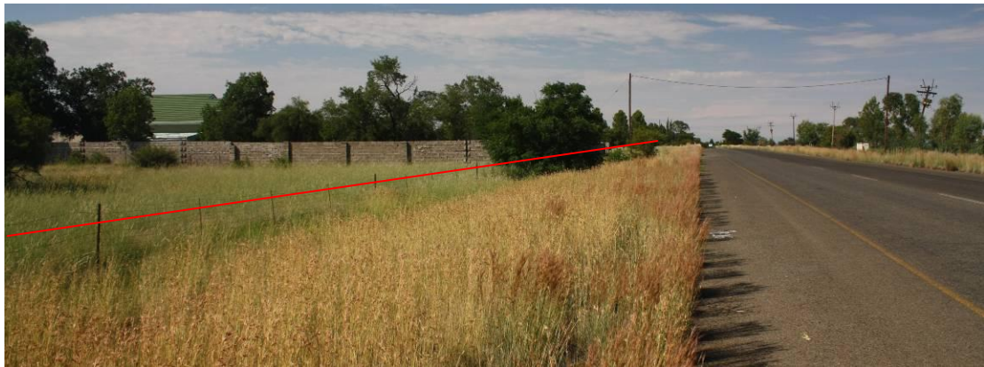
Figure 12: View of the Roodewal Small Holdings through which the pipeline will be installed (red line). This area is transformed.
