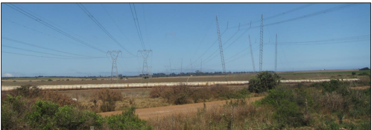
View towards the southeast in the middle of the power line route.
