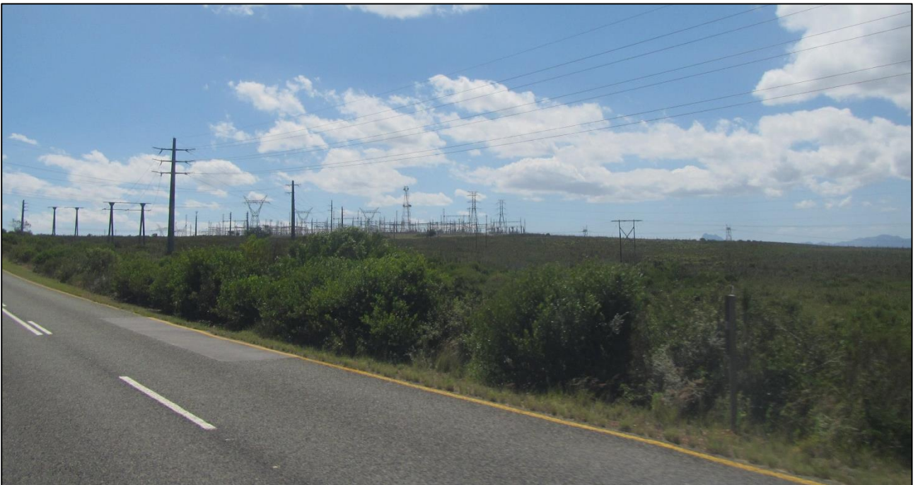
View towards the northwest along the powerline route to the substation at its north-western end as seen from the R327.
